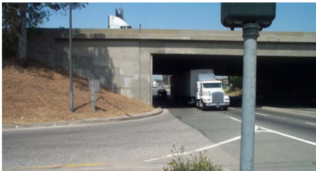
Ramp Entrance at Del Amo Blvd.
