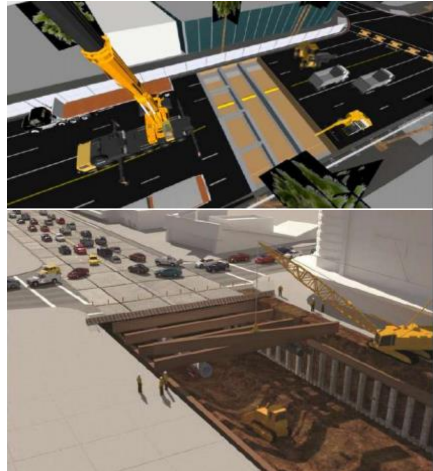
Renderings of typical street decking construction
