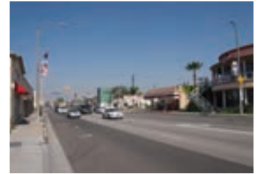
Figure 2-32 (Top) The Pioneer Station site in a broad ROW (Bottom) This terminus station can be catalyst for transit-oriented development and provides direct access to Artesia’s “Little India” on Pioneer Boulevard
