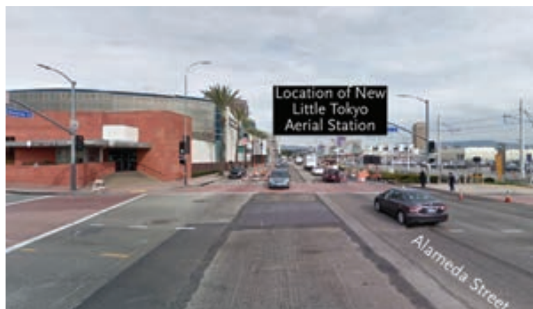
Figure 1-12: Proposed Little Tokyo/Arts District Station location at 1st/Alameda (looking north)
