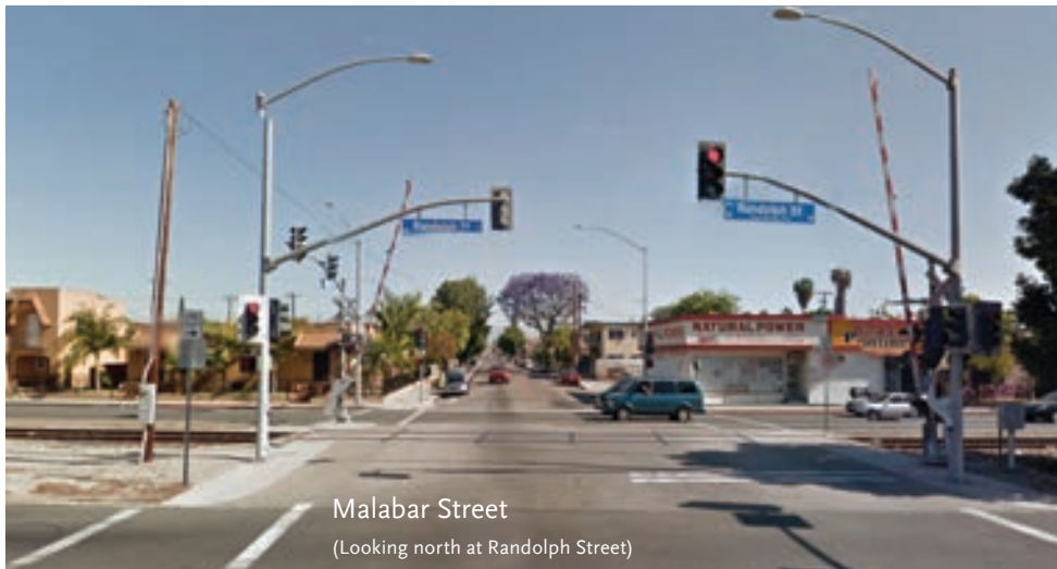
Figure 1-28: Malabar Street view
