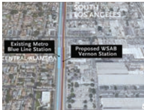
Figure 2-9: Vernon Station at the Metro Blue Line
