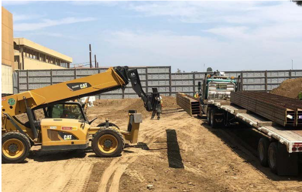
Unloading Steel Posts for Sound Wall at 1940 CPE
