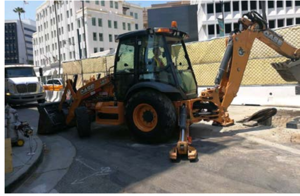
SCG Gas Pipe Excavation in Beverly Hills
