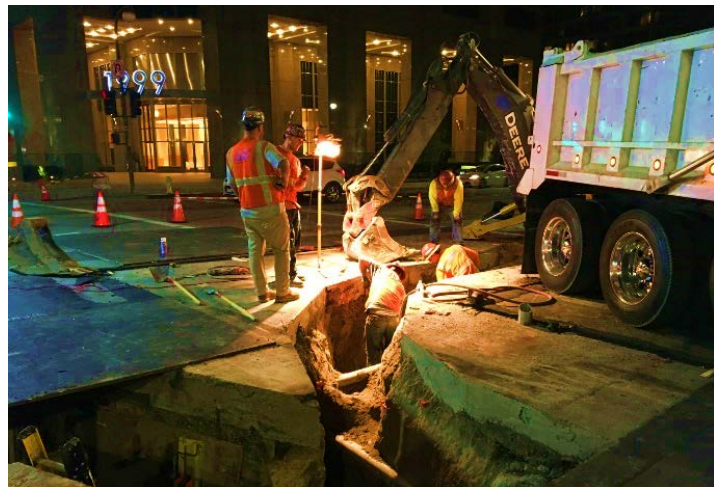
AT&T Utility Trench Work in Century City
