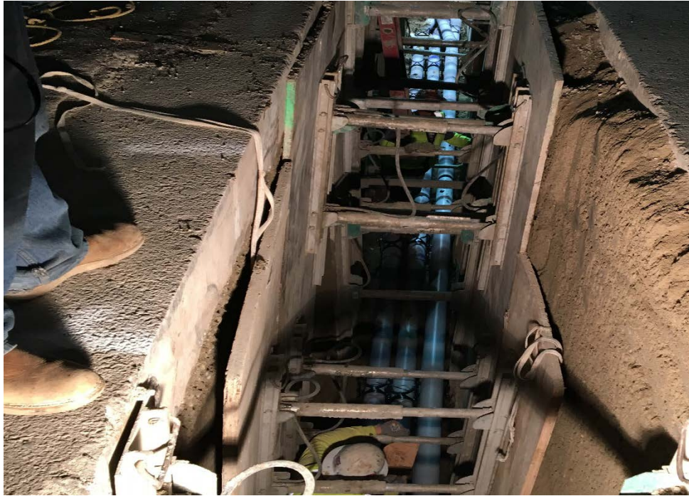
LADWP Power Utility Work in Century City
