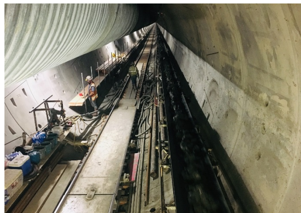
Reach 1 Tunnel Looking West
