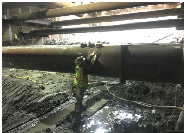
Strain Gauge Installation at Wilshire/La Cienega Station
