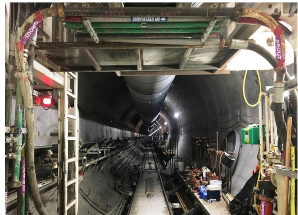
Reach 1 Tunnel Looking West
