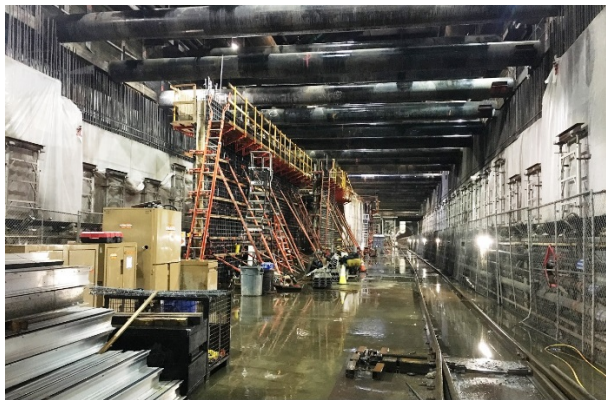
Wilshire/La Brea Station Looking East
