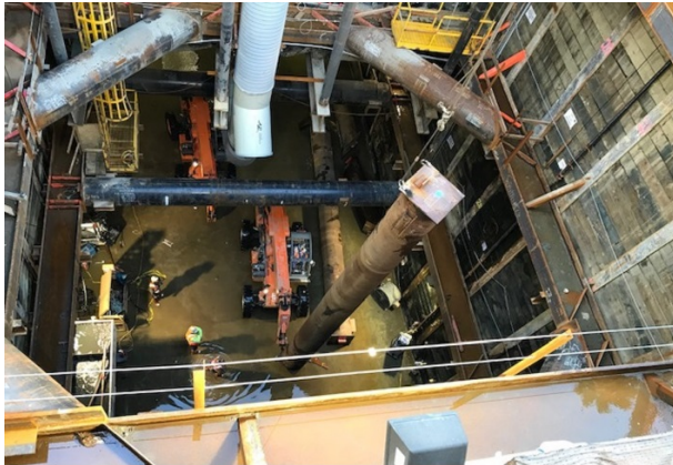
Lifting Strut out of the Wilshire/Western Shaft
