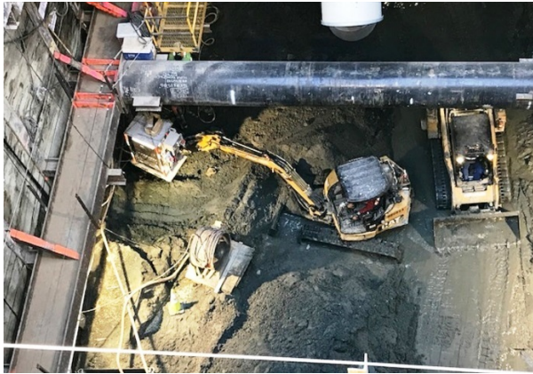
Excavation at Wilshire/Western TBM Retrieval Shaft
