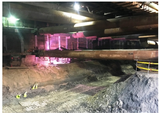
Welding Struts at Wilshire/La Cienega Station
