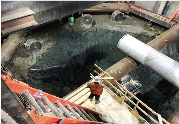
Excavation at Wilshire/Western
