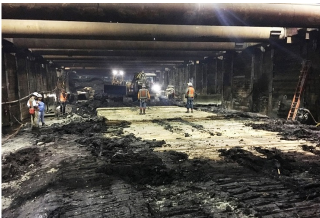
Crane Pads Set near Wilshire/Fairfax Subgrade
