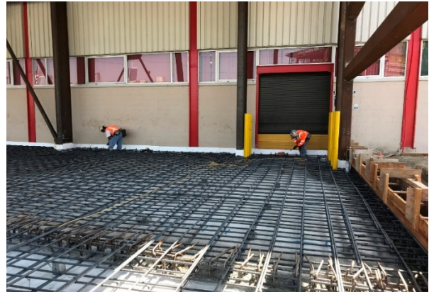
Division 20 Building – Slab on Grade Activities
