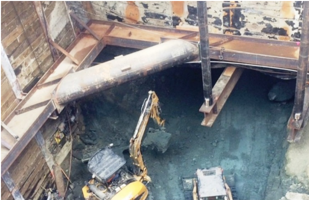
Excavation under the BRS at Wilshire/Western
