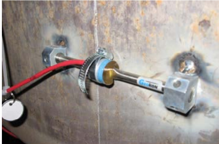
Exploratory Shaft Strain Gauge
