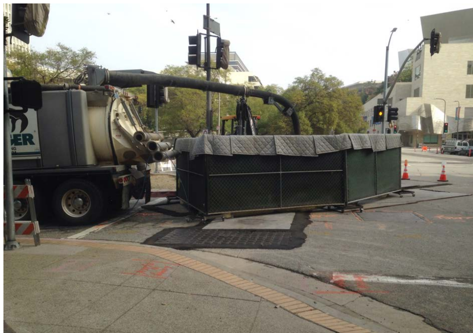
C0980 Contract – Potholing at 2 nd /Hope Sts.
