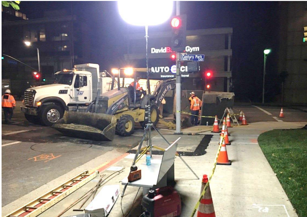
Century City Constellation Joint Trench
