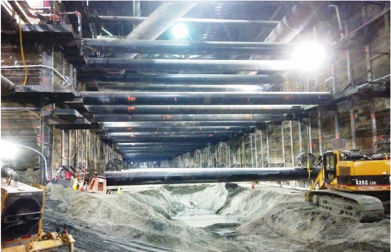
Under Deck Excavation at Wilshire/La Brea Station
