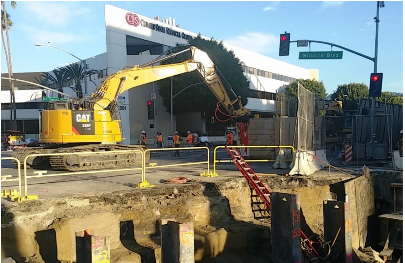
Decking Operation at Wilshire/La Cienega Station
