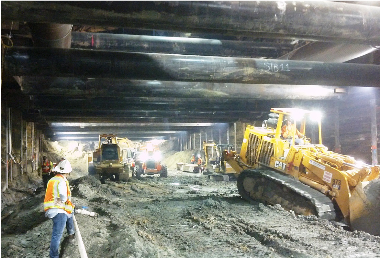
Under Deck Excavation at Wilshire/La Brea Station
