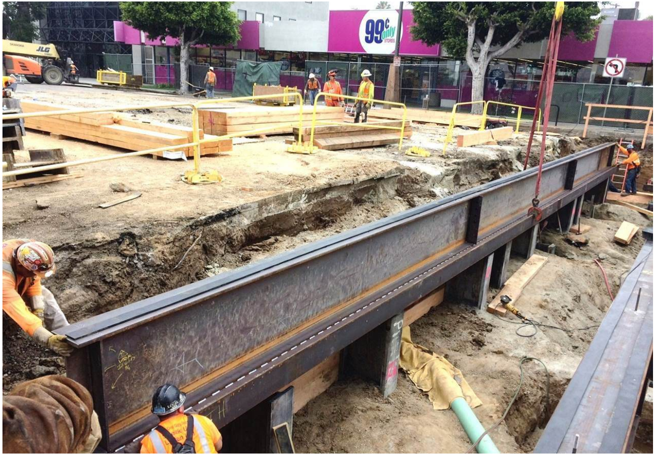
Wilshire/Fairfax Decking Operation in Progress
