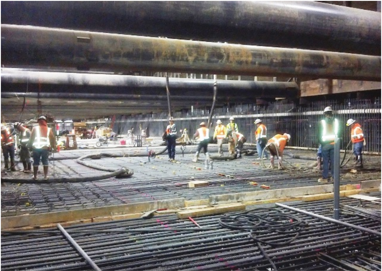
Wilshire/La Brea Station
