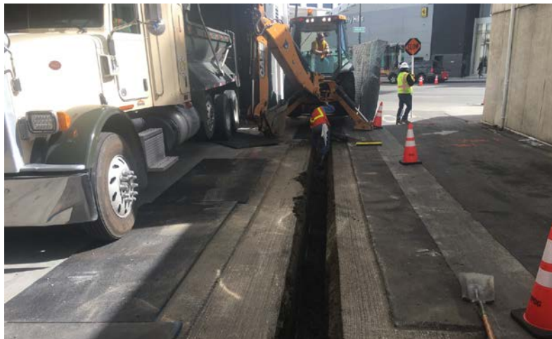
SCG Utility Work in Beverly Hills
