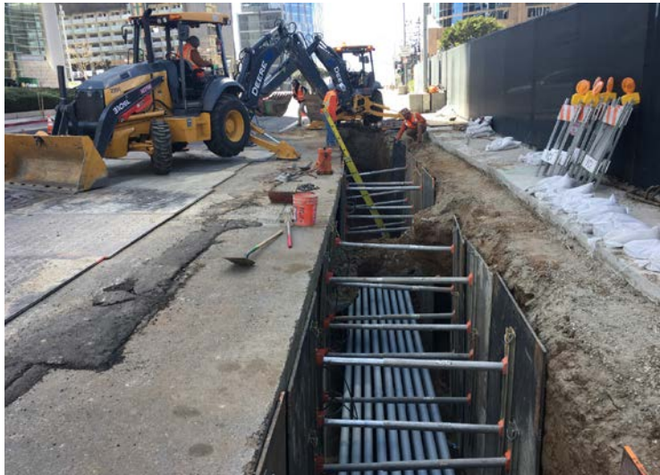
AT&T Conduit Installation in Century City
