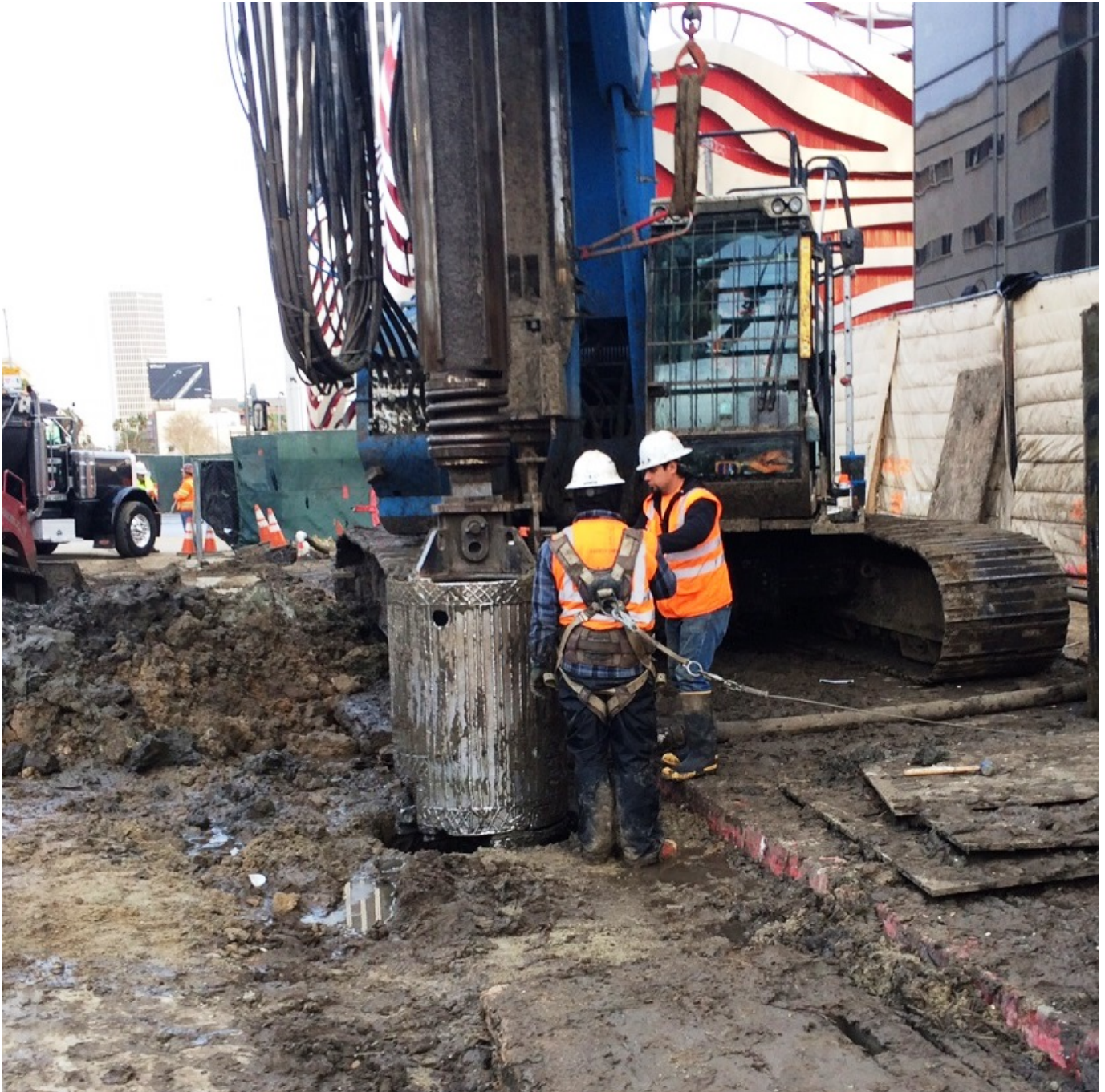
Wilshire/Fairfax Station Pile Installation Activities
