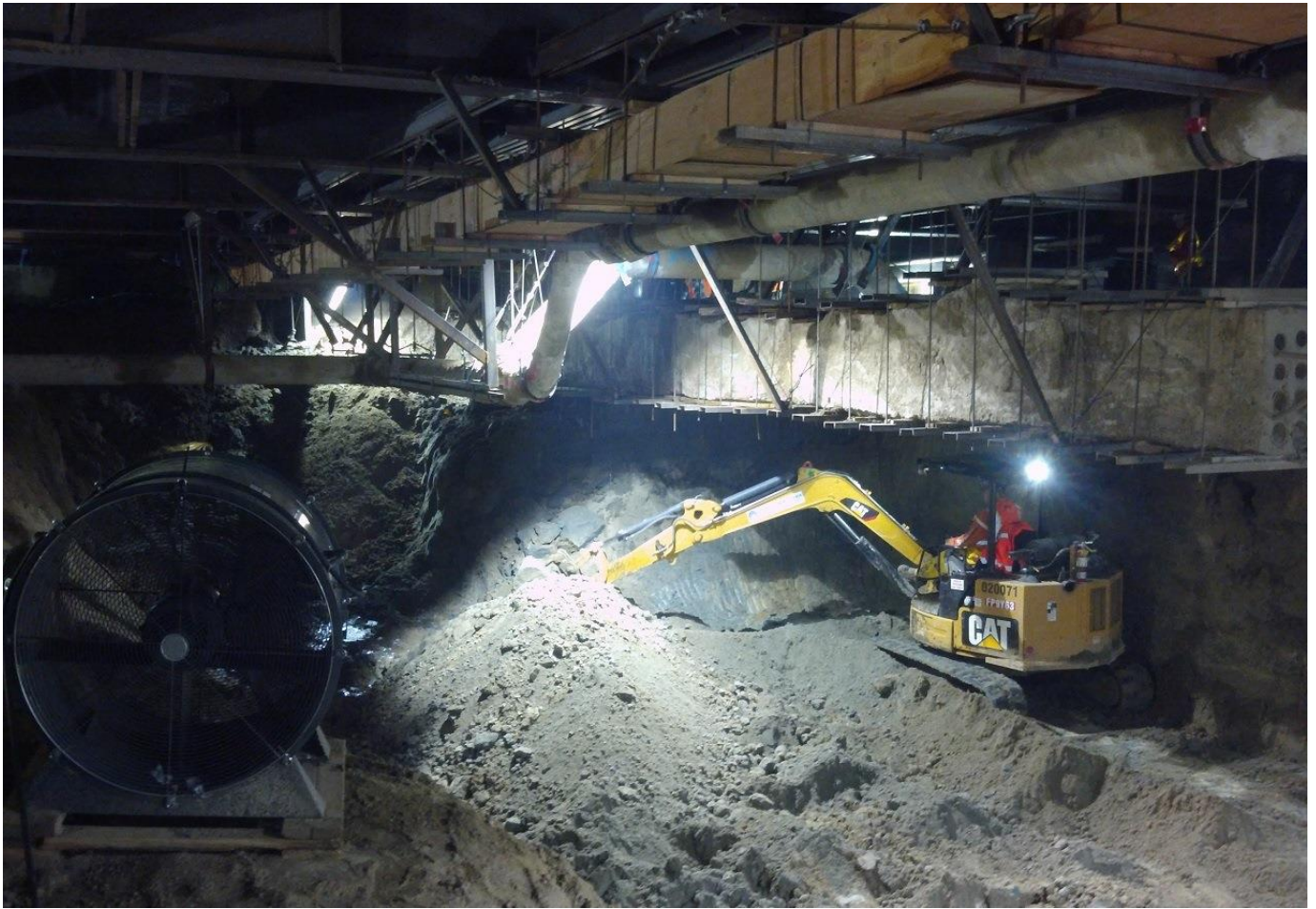
Wilshire/La Brea Station Excavation under Decking
