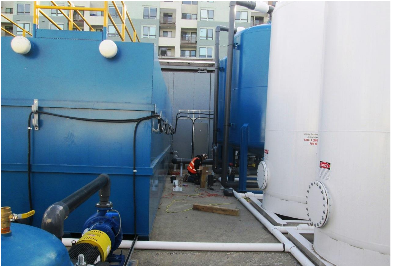
Installation of Water Treatment System at South Wilshire/La Brea Yard
