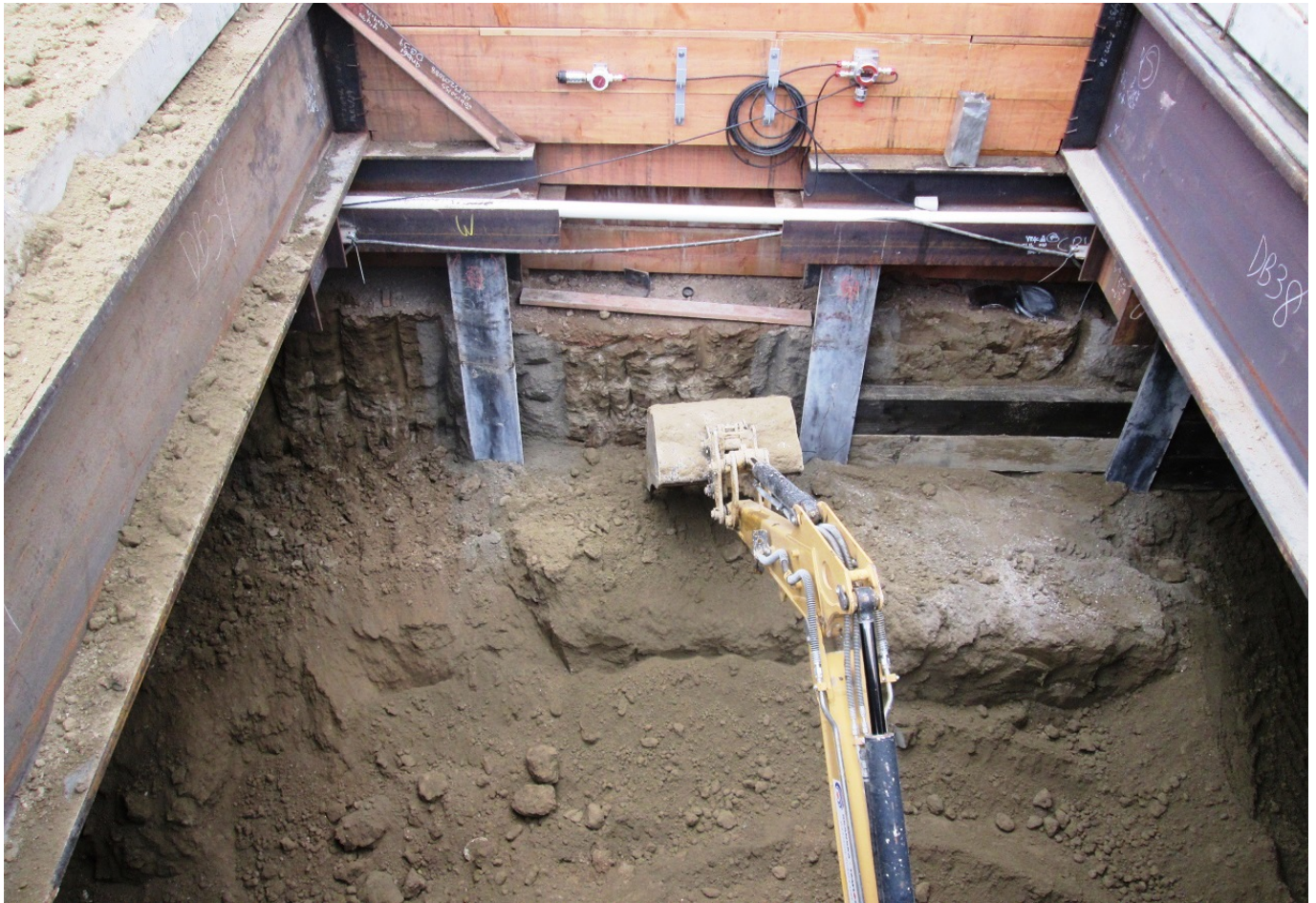
Wilshire/La Brea Station Excavation
