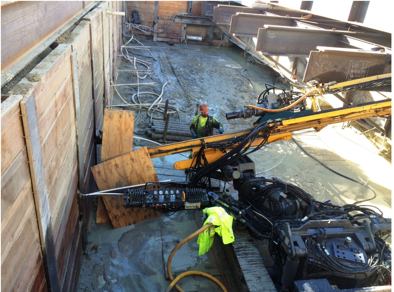
Wilshire/La Brea South Muck Shaft Tieback Grouting
