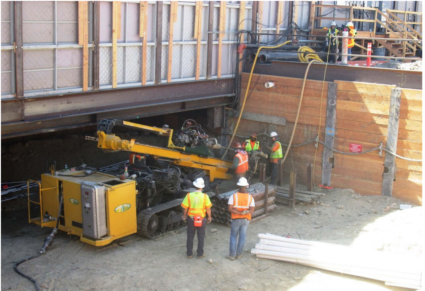
Wilshire/La Brea North Muck Shaft Tieback Installation
