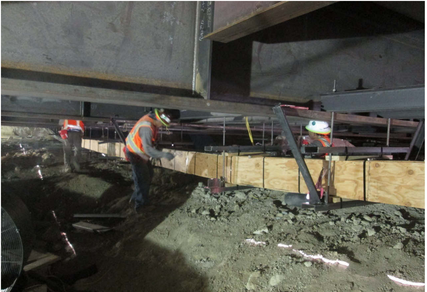
C1045 Contractor Hanging in Place Telecommunications Duct Bank under the Street Decking at Wilshire/La Brea Station
