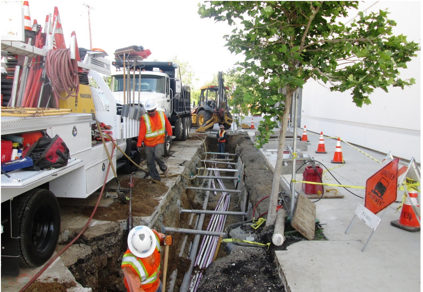
C1045 Contractor Relocating Telecom Conduits on Sycamore North of Wilshire Boulevard
