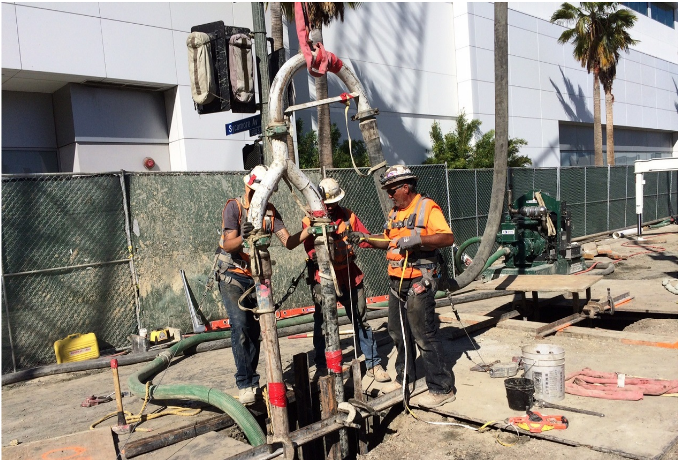
C1045 Contractor Placing Concrete on Pile #78 at the Wilshire/La Brea Station
