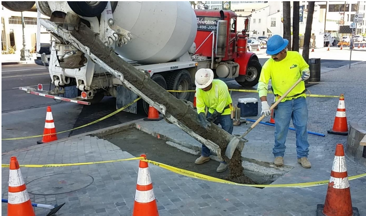
C1056 Contractor Restoring Sidewalk over Southern California Edison's Ductbank East of La Cienega Boulevard
