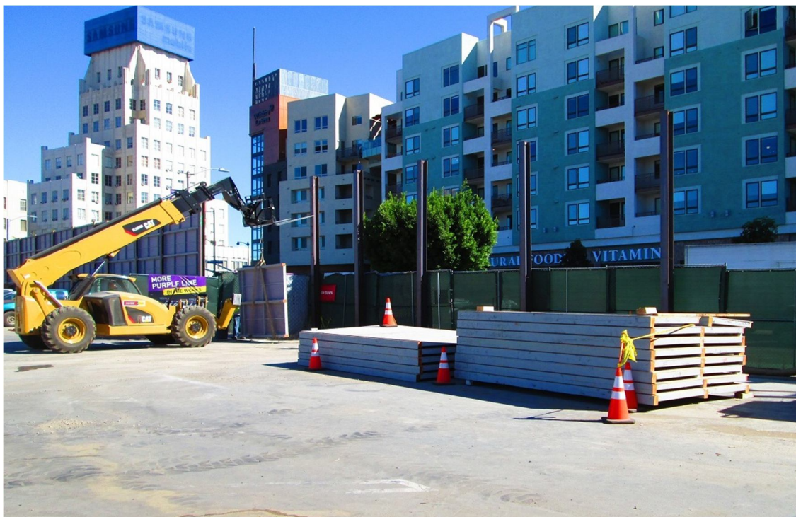
C1045 Contractor Installing Soundwall Panels at the South Wilshire/La Brea Construction Staging Site
