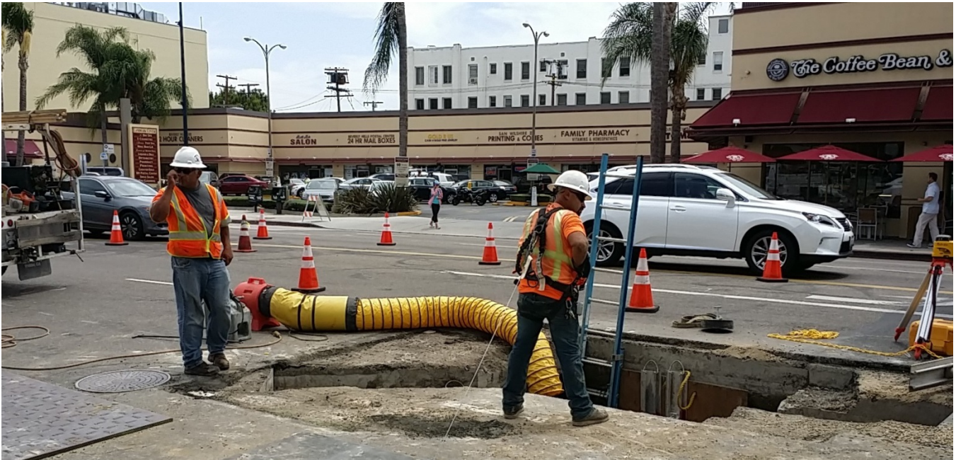
C1056 Contractor Relocating Utilities along Wilshire Blvd. Westbound Lanes
