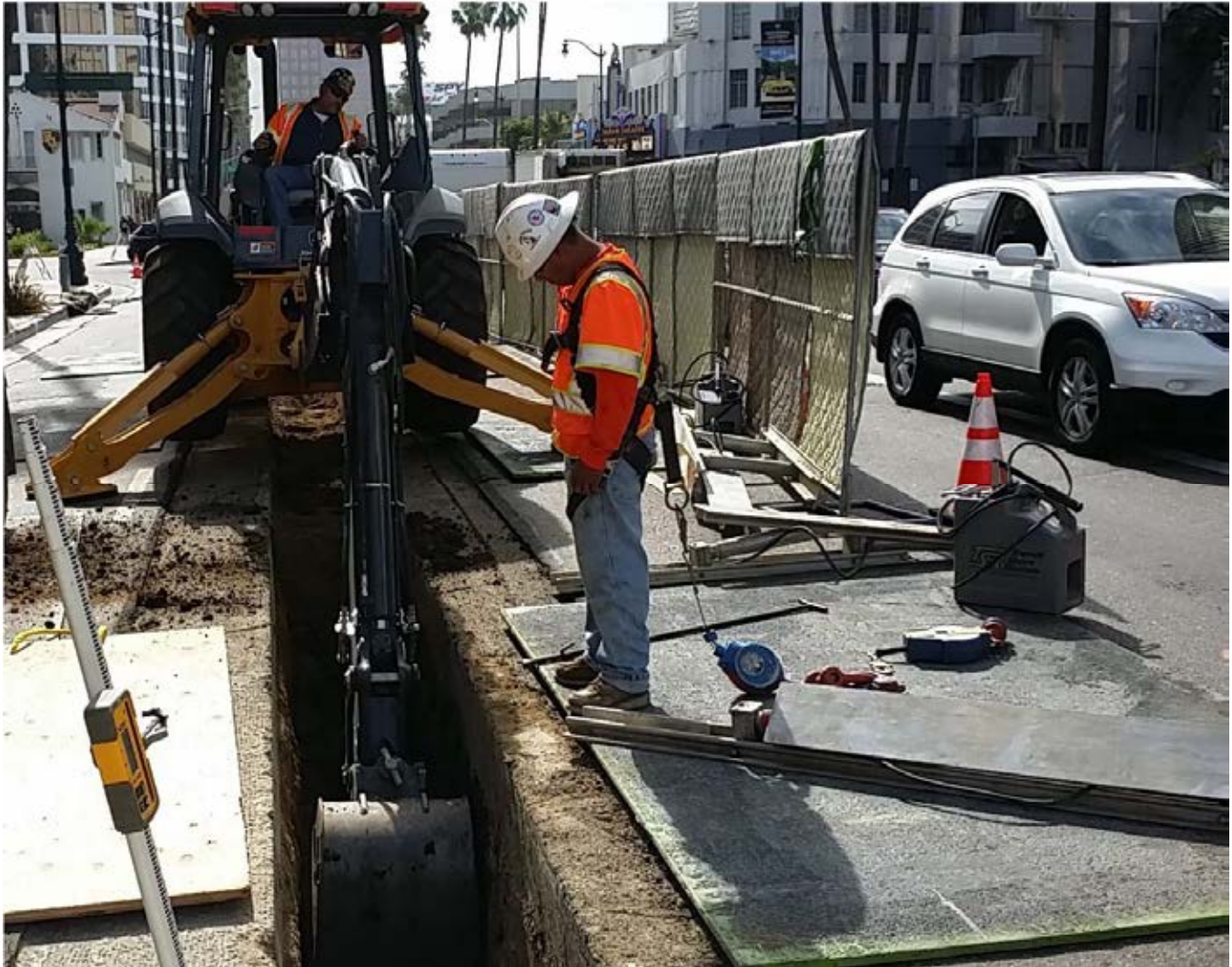
C1056 Wilshire/La Cienega AUR Contractor Excavating SCE Power Ductbank East of La Cienega Boulevard
