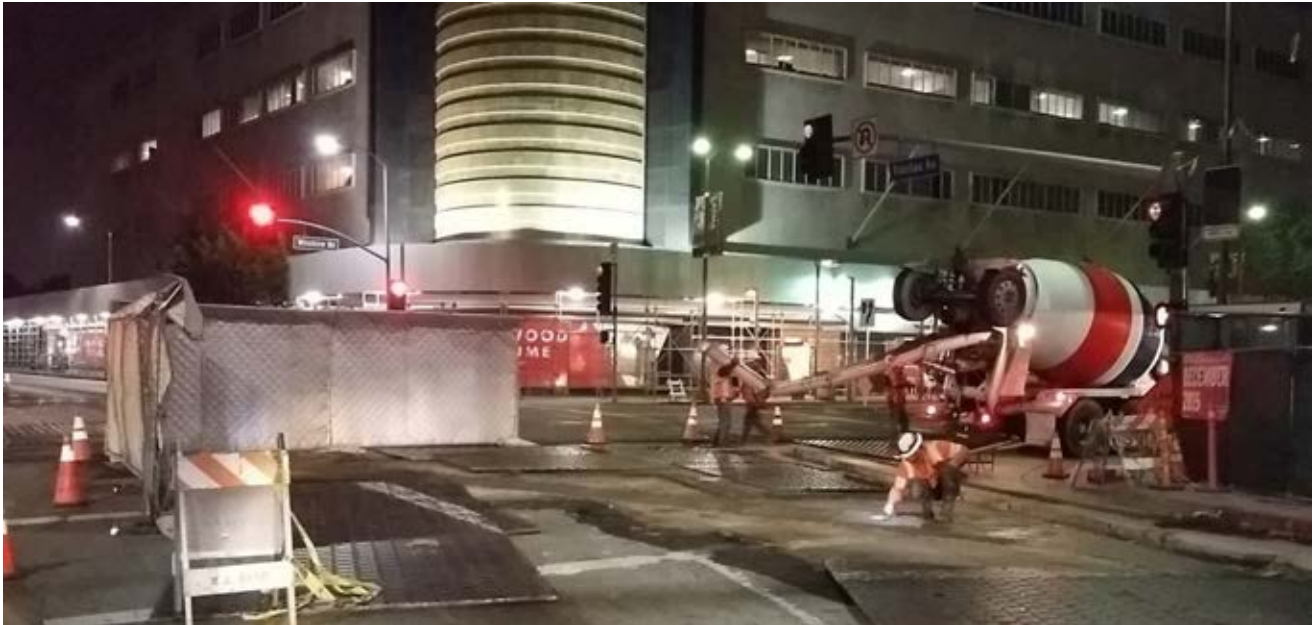
C1055 Wilshire/Fairfax AUR Contractor Restoring Pavement for Power Trenches at Wilshire/Fairfax Intersection
