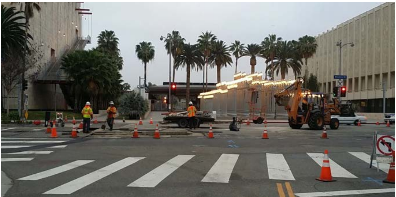
C1055 Wilshire/Fairfax AUR Contractor Completing Water Line Relocation at Wilshire/Ogden
