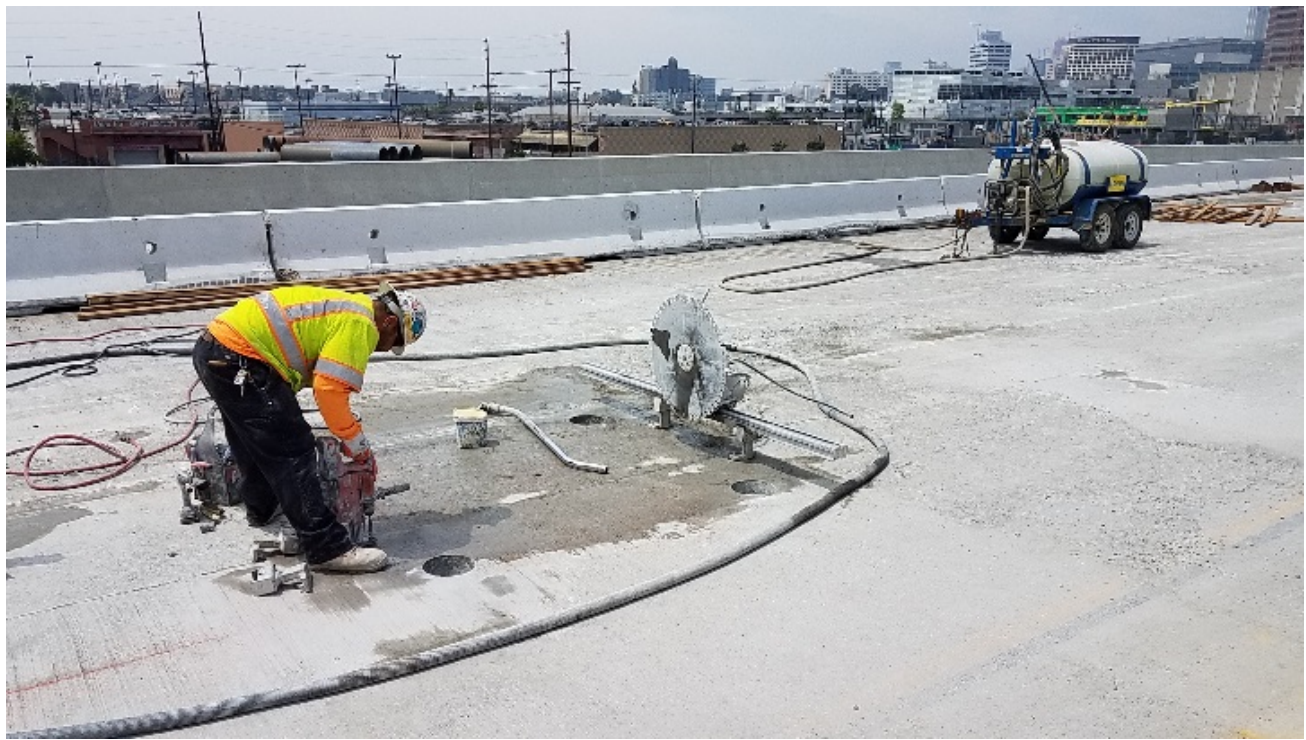
Cutting stair opening in deck.
