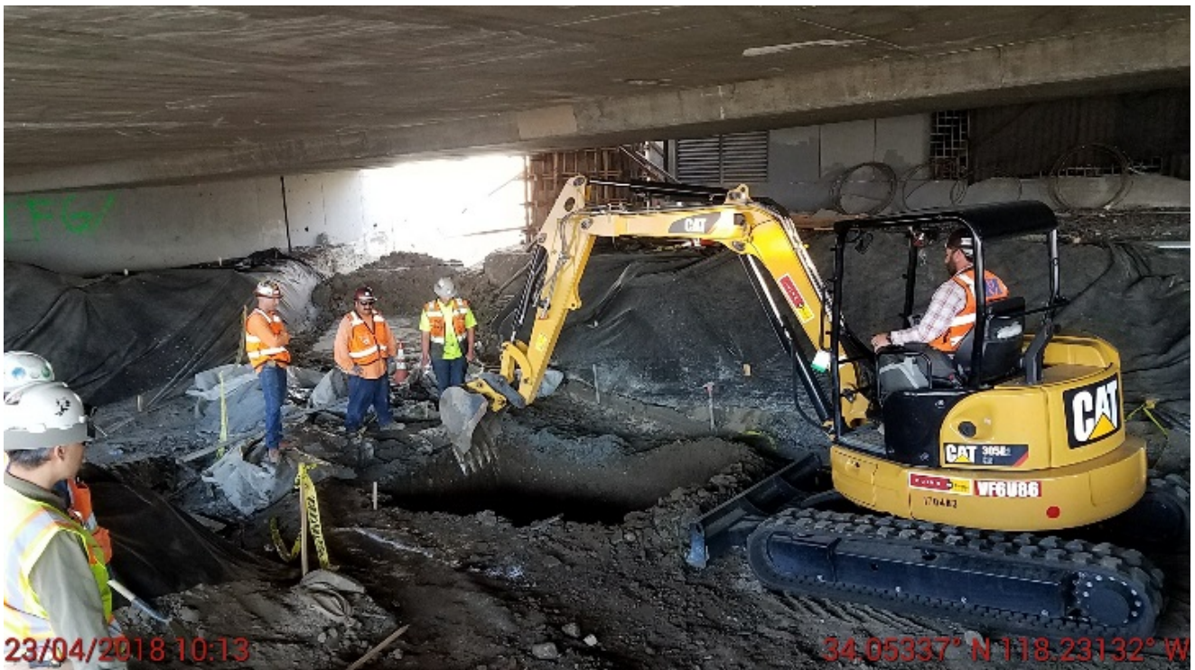
Micropile excavation.
