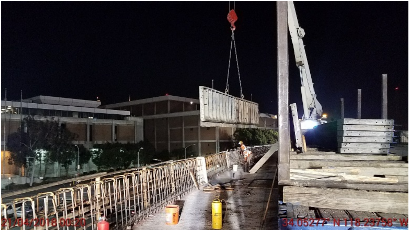
Setting forms for left side for 2 nd pour.
