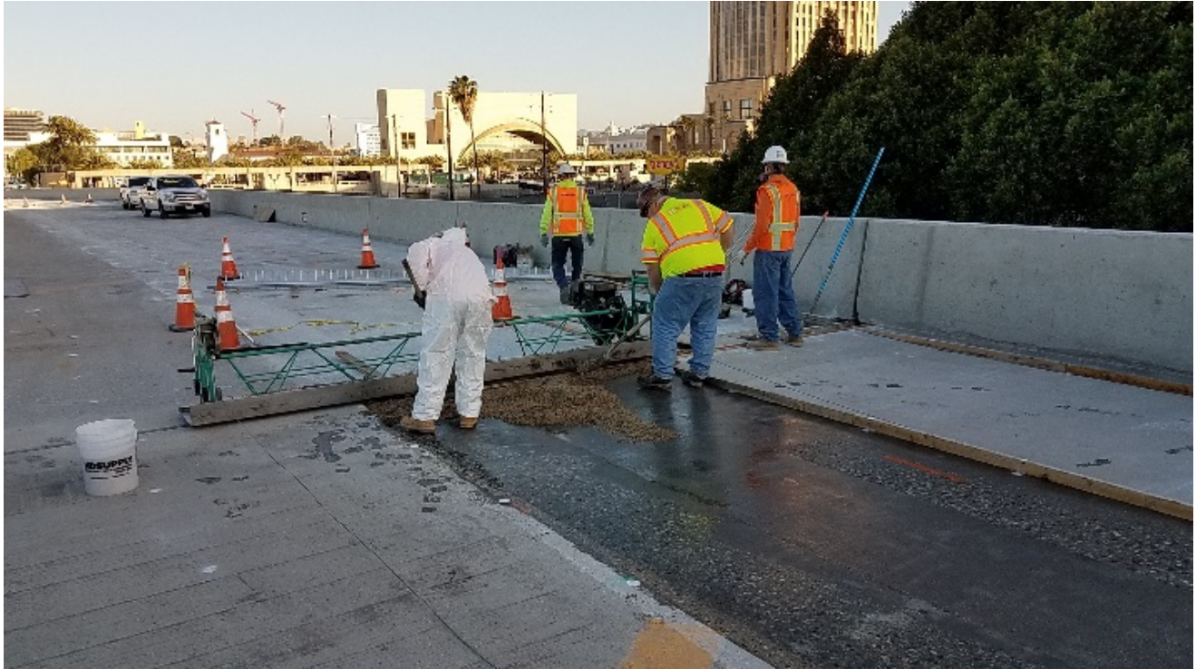
Polyester concrete overlay.
