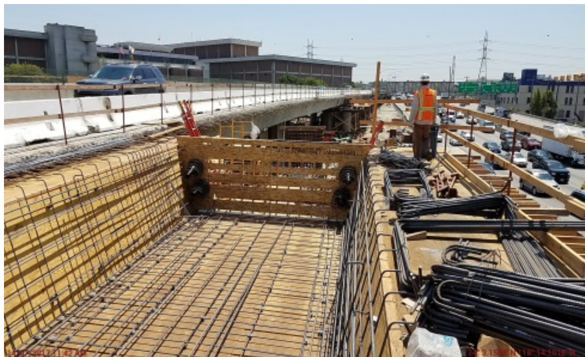
Frame 1 soffit/stem rebar installation.
