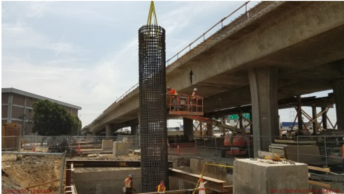
Column cage at Bent 6.
