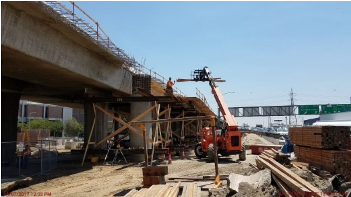
Frame 3 Falsework installation.
