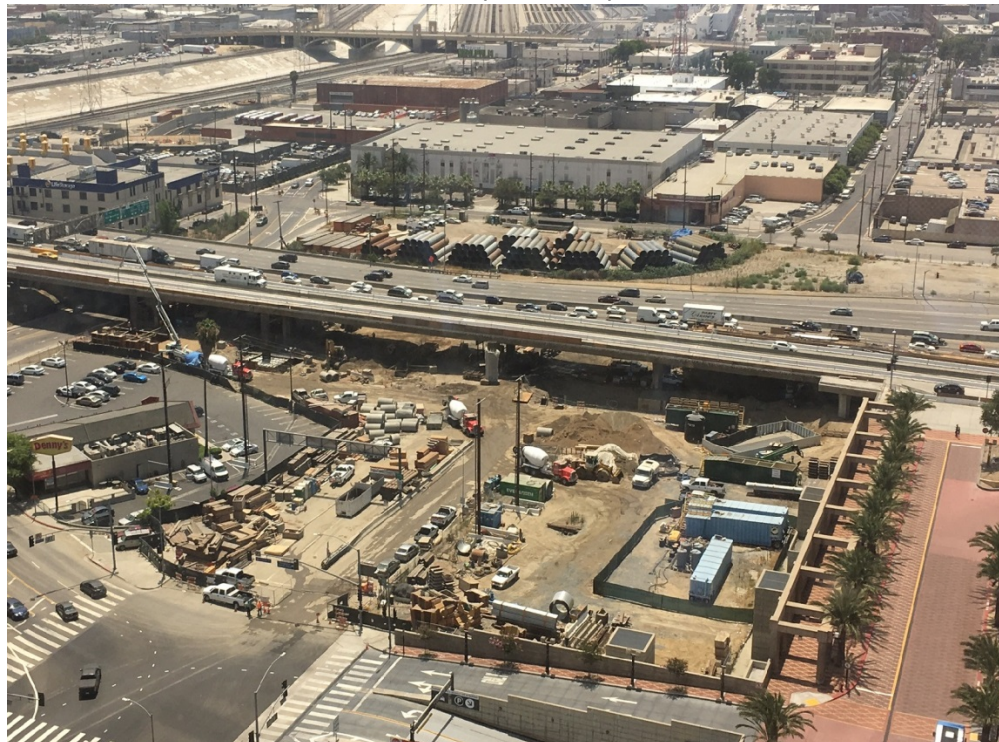
AERIAL PHOTOGRAPH OF JOBSITE (6-30-2017)
