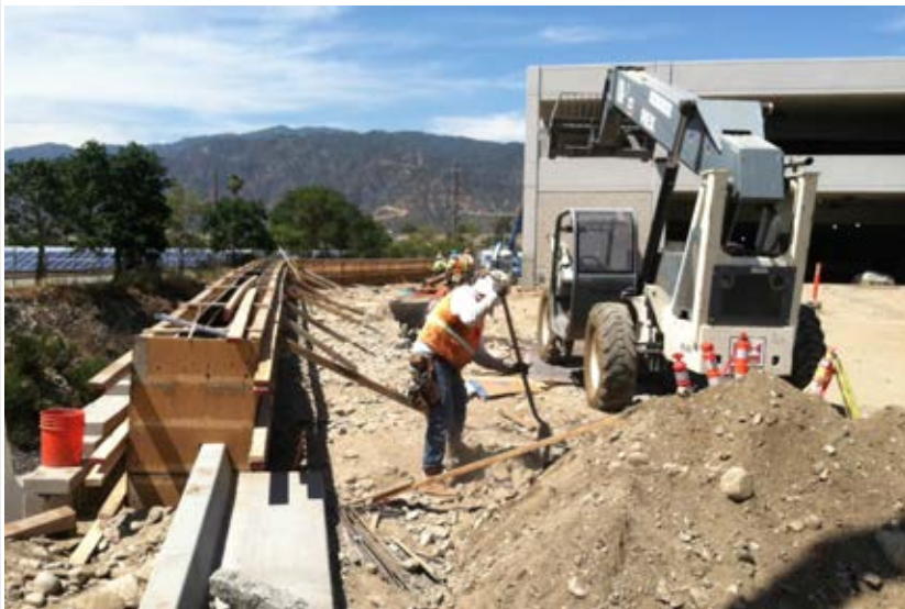
Irwindale Parking Structure Site Work
