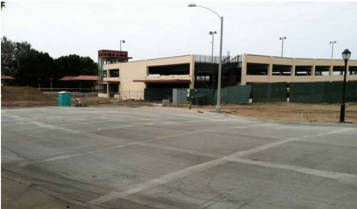
Monrovia Parking Structure Site Overview
