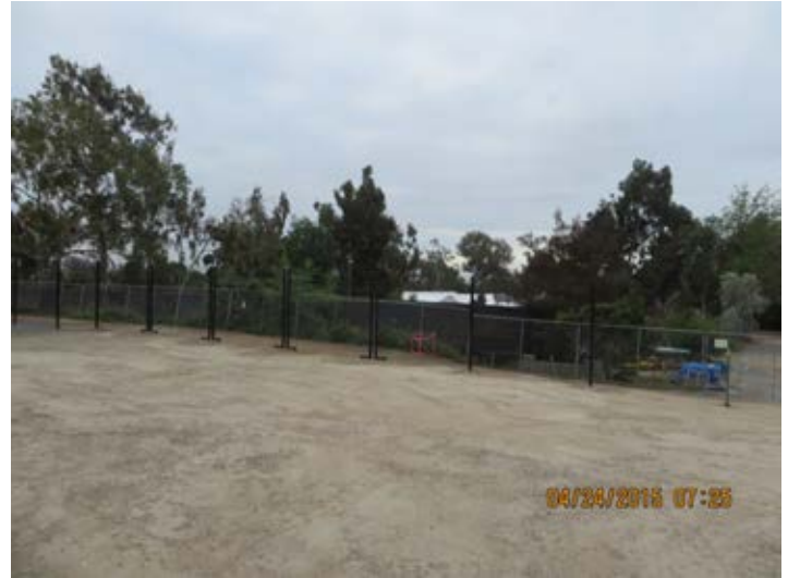
Segment 1: Baldwin TPSS Wire Mesh Fence
