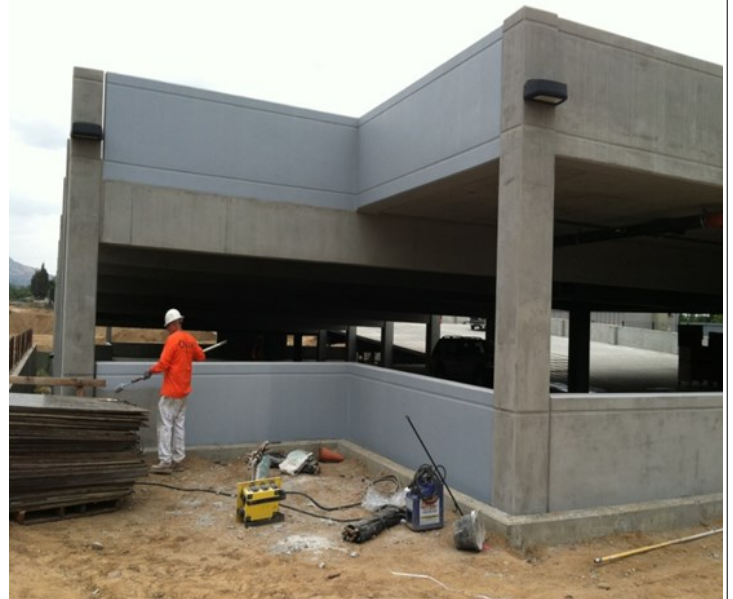
Azusa-Citrus Parking Structure Paint Work
