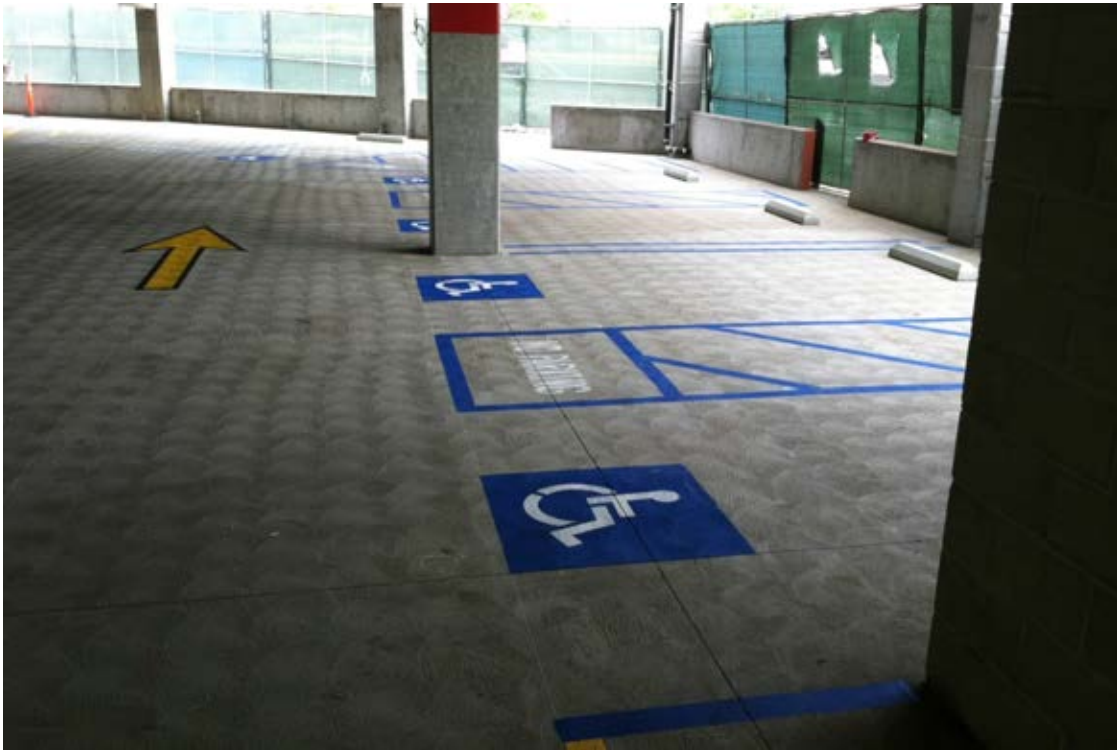
Arcadia Parking Structure Striping
