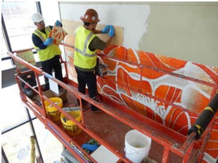
Operations Campus: Work on Lobby Art Wall
