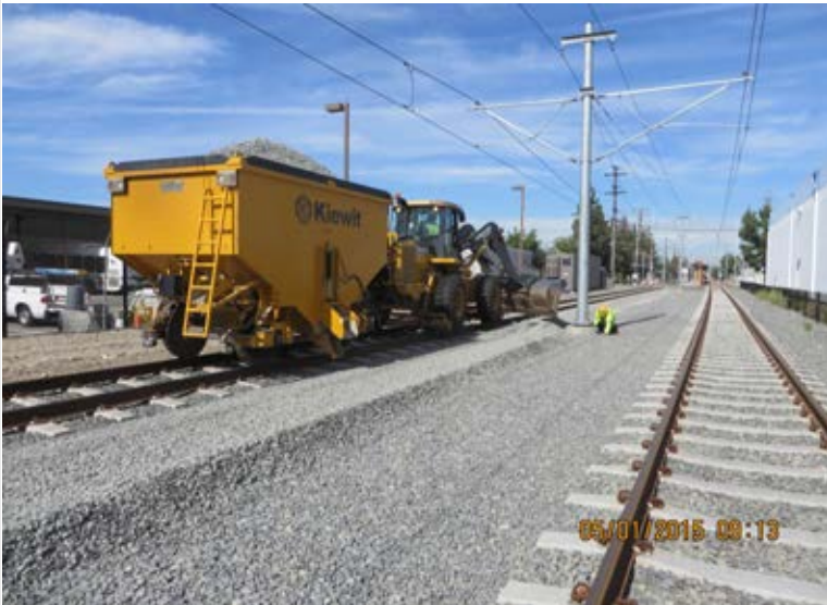
Segment 3: Walkway Ballast Placement
