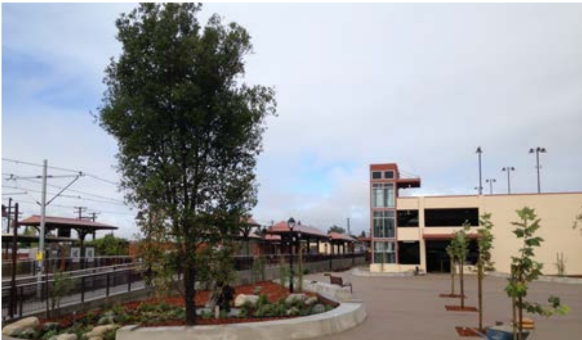
Monrovia Parking Structure Site Overview
