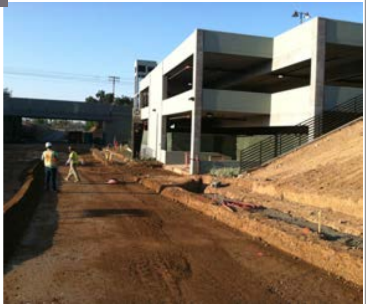
Azusa-Citrus Parking Structure Site Overview
