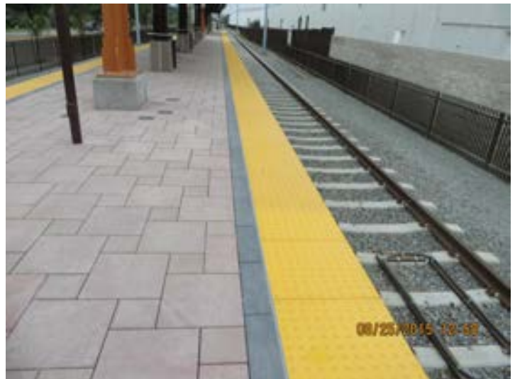
Segment 3: Duarte Station - Dielectric Caulking
