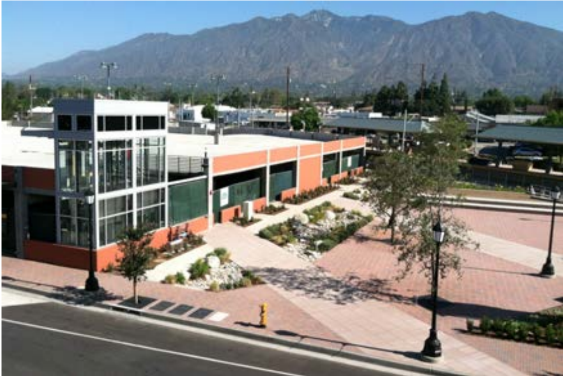
Arcadia Parking Structure Site Overview
