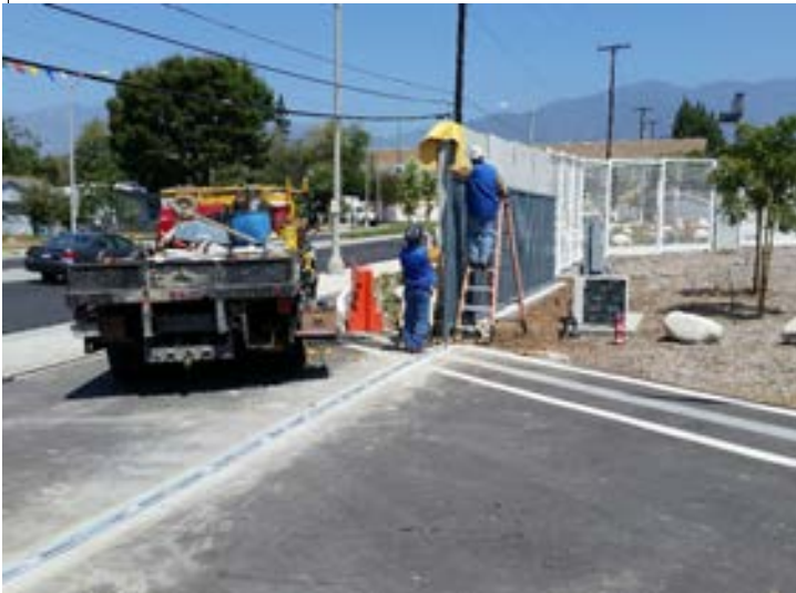
Operations Campus: Main Gate Final Adjustments
