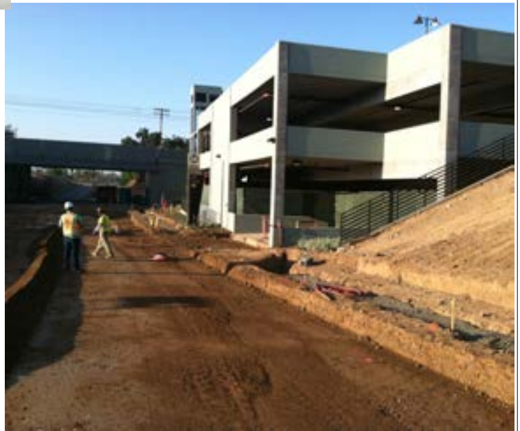
Azusa-Citrus Parking Structure Site Overview
