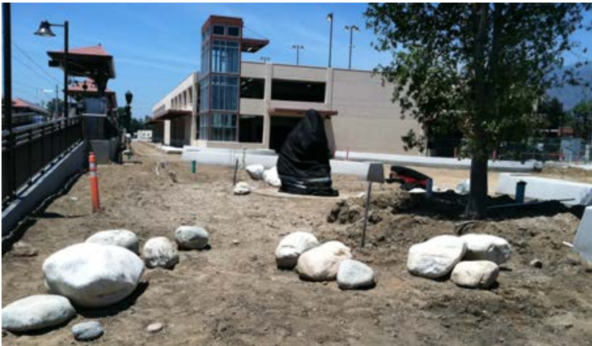
Monrovia Parking Structure Site Overview
