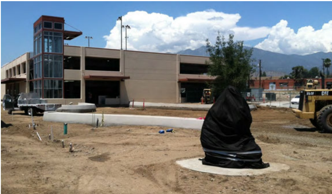
Monrovia Parking Structure Site Overview
