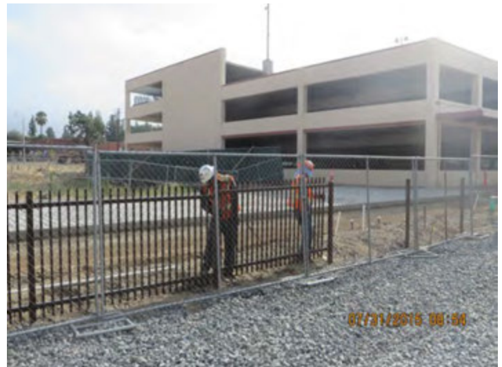
Segment 3: Monrovia Station - Picket Fence Installation
