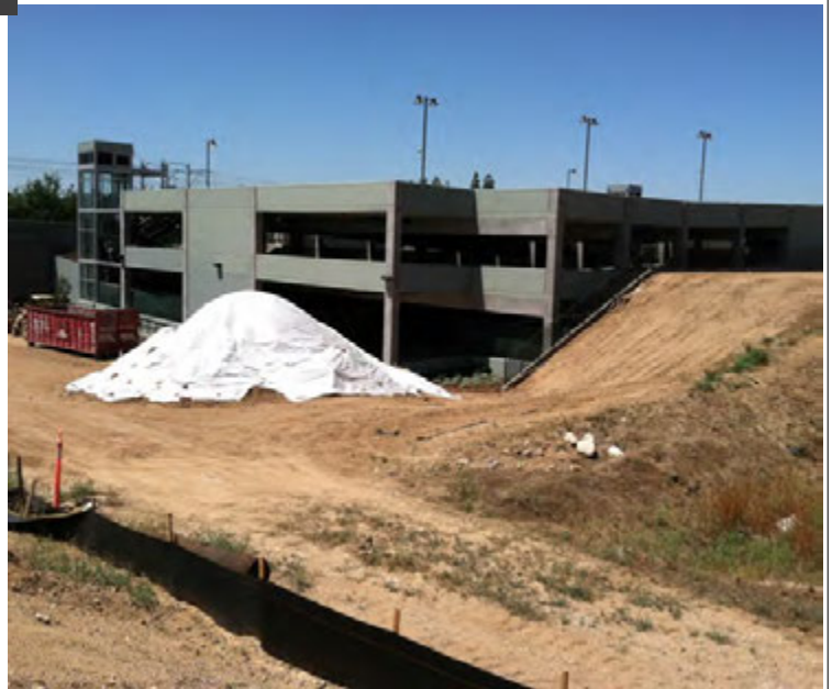
Azusa-Citrus Parking Structure Site Overview
