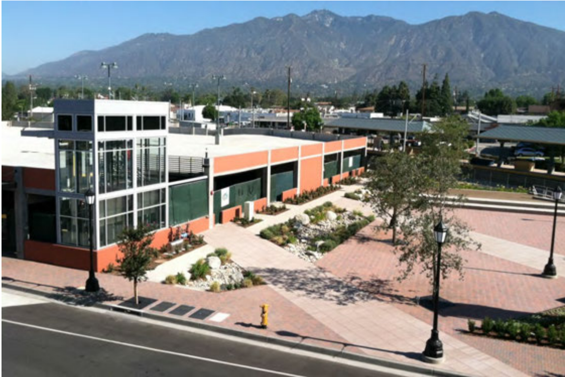
Arcadia Parking Structure Site Overview
