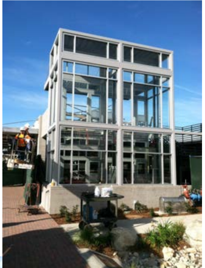
Arcadia Elevator - Glass Installation Complete
