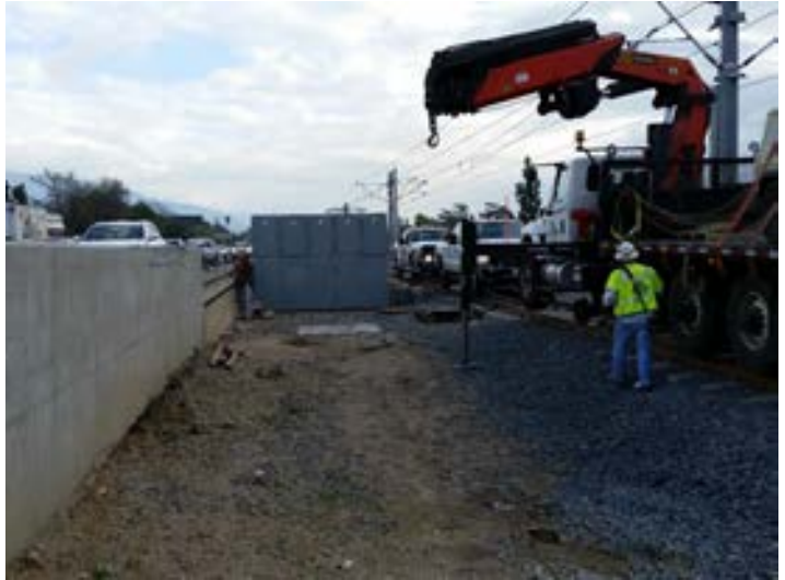
Segment 1: Michillinda TPSS Cabinet Installation
