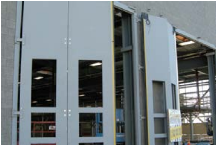
Operations Campus: Bi-fold Train Doors at Paint Shop being installed
