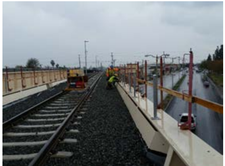
Segment 4: Foothill Bridge Cable Installation
