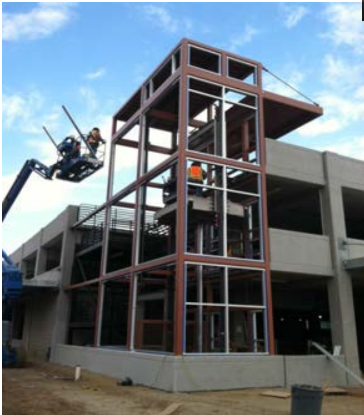
Monrovia Elevator - Steel Framing Installed
