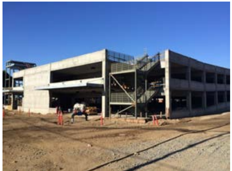
Monrovia Parking Structure Site Overview
