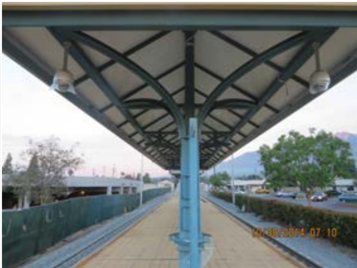
Segment 2: Arcadia Station Light and Camera Fixtures Installed
