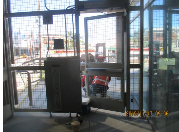
Hardware and doors work under progress at Trans. Level 1.
