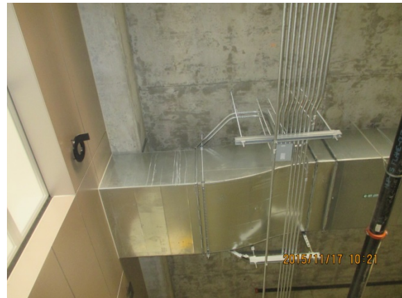
Water Leaking from storm drain connection at Parking Bldg. L1.
