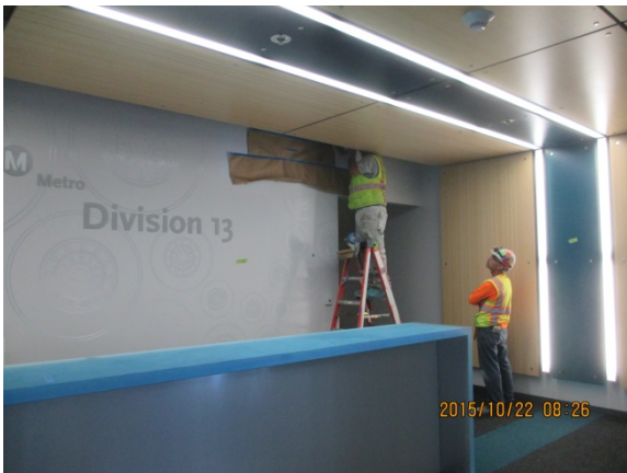
Changes in progress at Transportation Bldg. Level 2.
