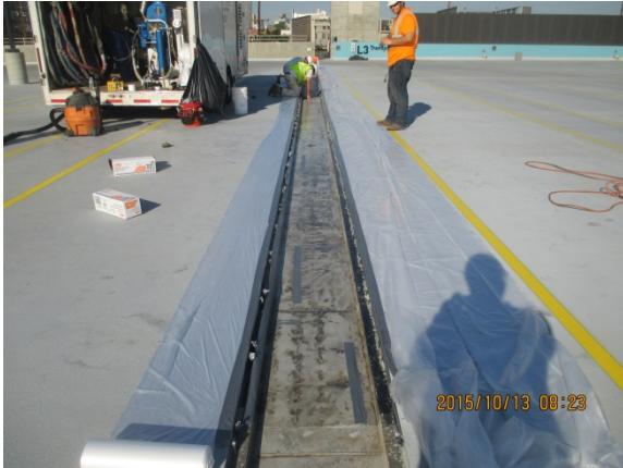
Trench drain repairs commenced at Upper Level Roof Parking Bldg.
