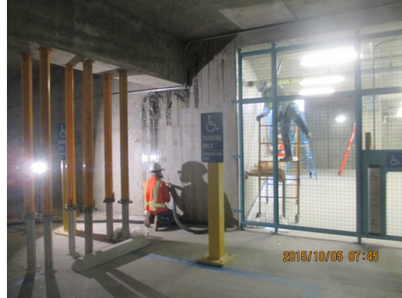
Crack repairs in progress at lower level of Parking Garage.
