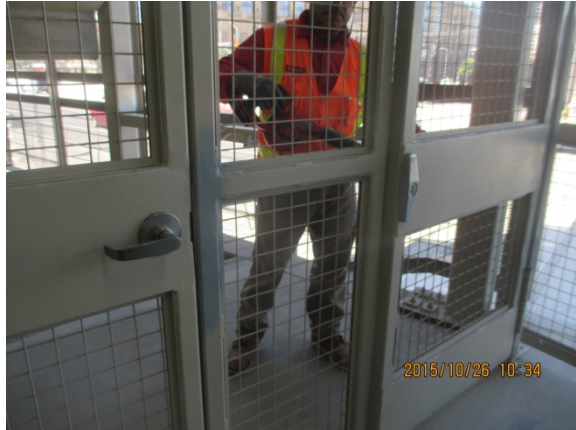
Hardware door work in progress at Transportation Bldg. Lvl 1.
