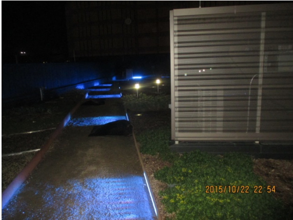
Night version of Vegetated Green Roof.
