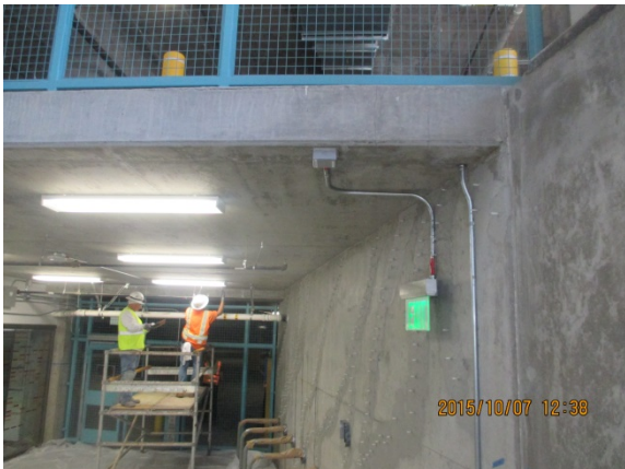
Installation of light fixtures in progress at Trans. Bldg. L.
