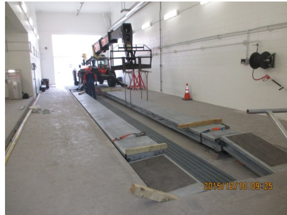
Preparation for chassis wash lift installation.
