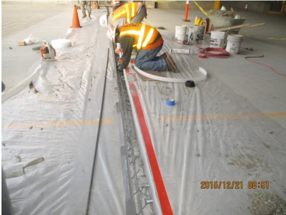
Repair of concrete slab crack.
