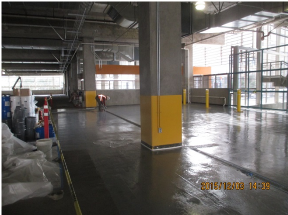
Parking Garage level 1 finishing layer.
