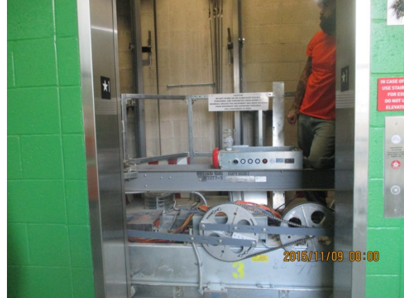
Elevator 3 work under progress at Maintenance Bldg. Level 1 North.
