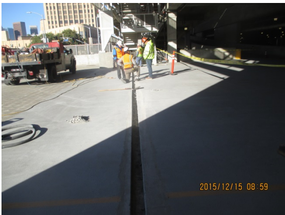
Repair of concrete slab crack.
