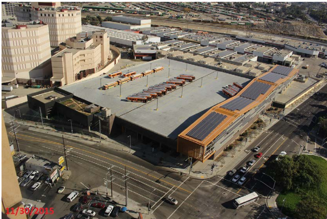
FLY OVER JOBSITE PHOTOGRAPH (11-30-2015)
