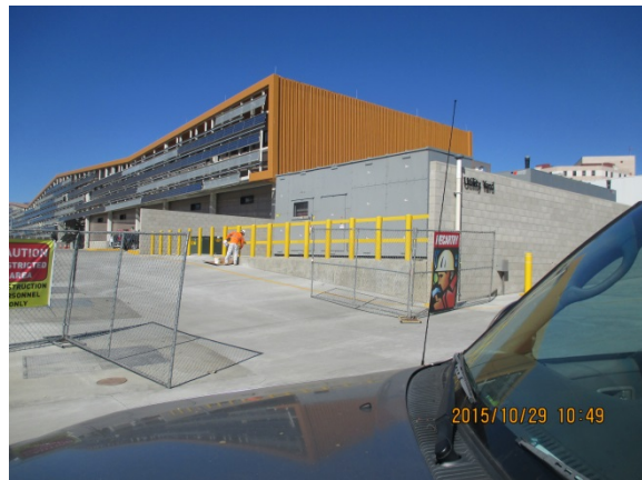
Painting of bollards in progress at Utility Yard Area.
