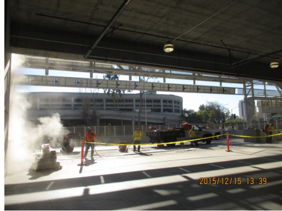
Cleaning before repair.
