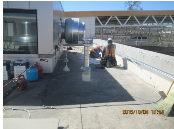
Leaking repairs in progress at Maintenance Bldg. Roof.
