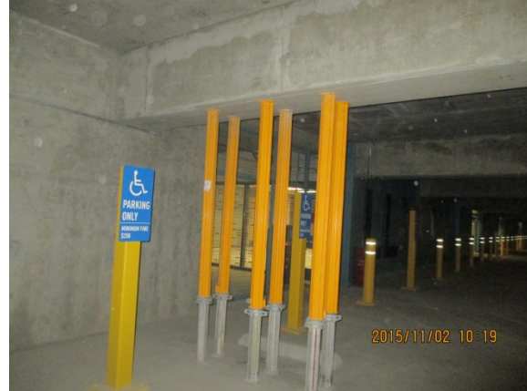
ADA and Beam supports re-design done at LL Parking Garage.
