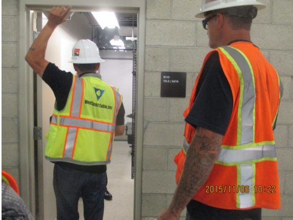
West Coast Cable Inc. at location for Tele/Data work.
