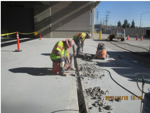
Trench created to repair crack.
