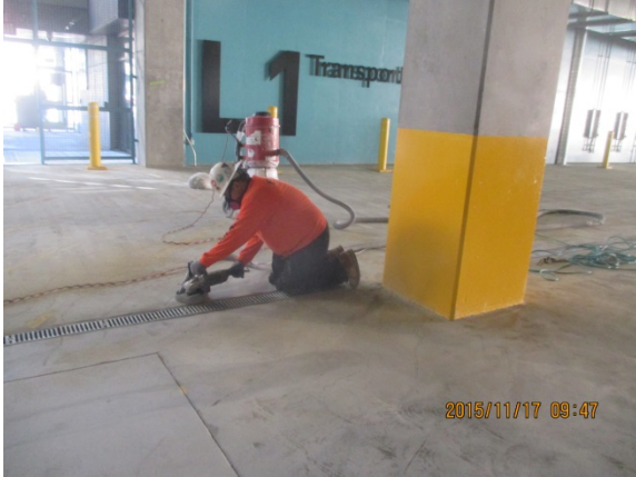
Concrete Finish work under progress at Parking Gar. Bldg. L1.
