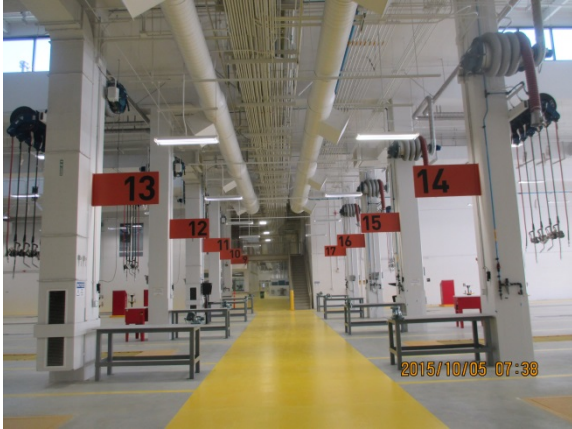
Striping work completed at Maintenance Bldg. Level 1.
