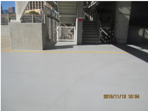
Concrete Slab crack repair completed and painted at Parking Bldg.
