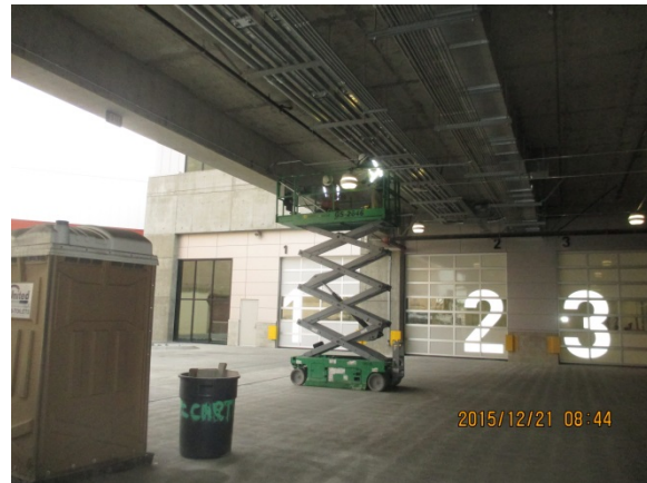
Lift to repair pipes.
