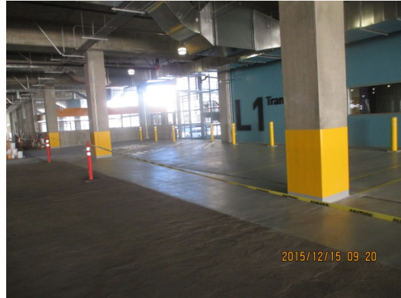
Stripping at level 1 parking garage.
