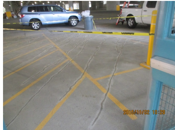
Crack testing and fixing on Parking Garage building in progress.
