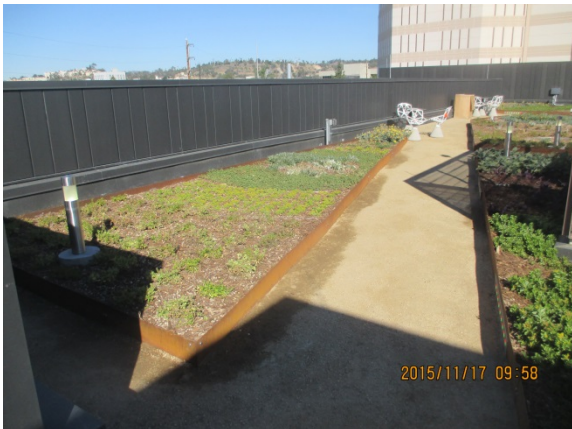
Vegetated Roof re-planting and cleaning completed and done.
