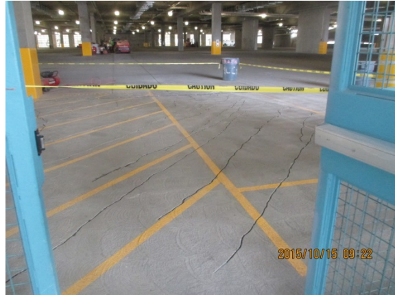
Sealing concrete deck at Level 1 Parking Garage Bldg.
