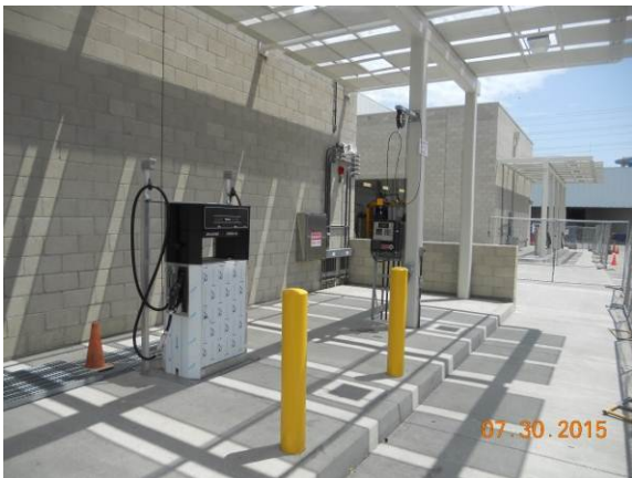
Fuel pump installation in progress at Non-Rev Fuel Area.
