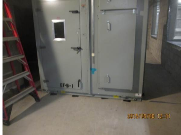
Power Panels installation for Exhaust Fans at Bldg. B Lower Level.
