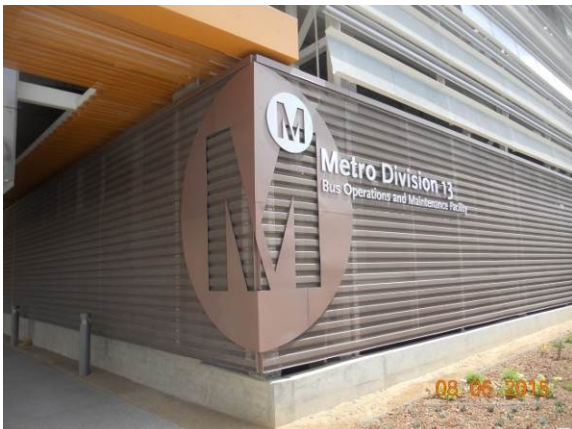
Metro Signage Installation completed at Southwest corner of Div 13.
