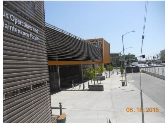
Street Tree planting & landscaping completed along Vignes St.
