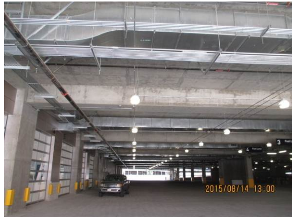
Column painting & lighting completed at Parking Bldg. Level 1.f.
