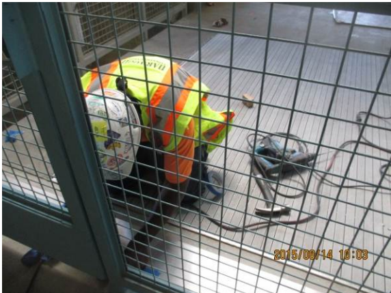
ADA Compliant Hinged Alum cover plate installation at Bldg A L1.
