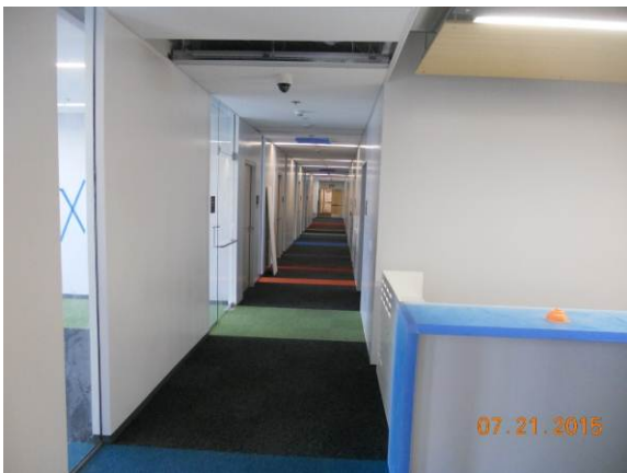
Carpeting & painting completed at Transportation Bldg. Level 2.
