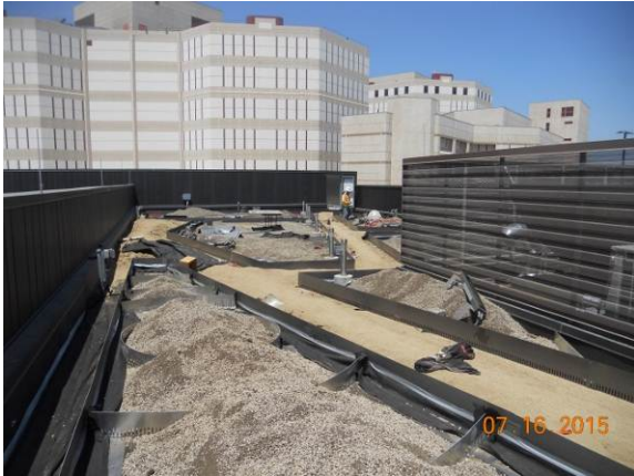
Vegetated Roof Garden Landscaping work in progress
