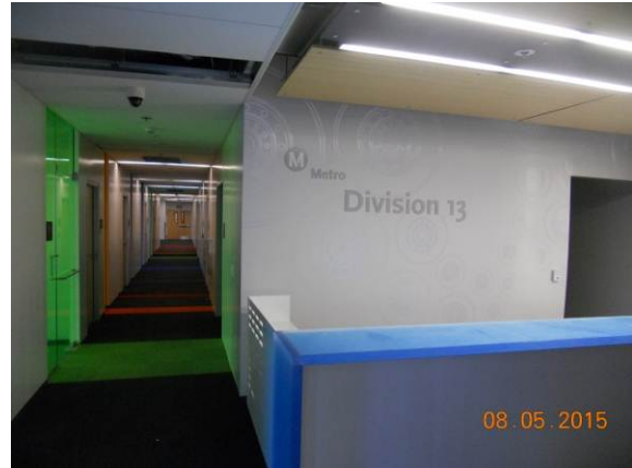
Painting, Carpeting and finishing now completed at Bldg. A L2
