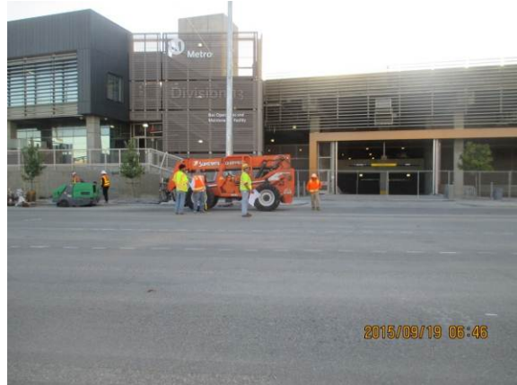
Vignes St Striping Prep, Layout & Lane opening in progress.
