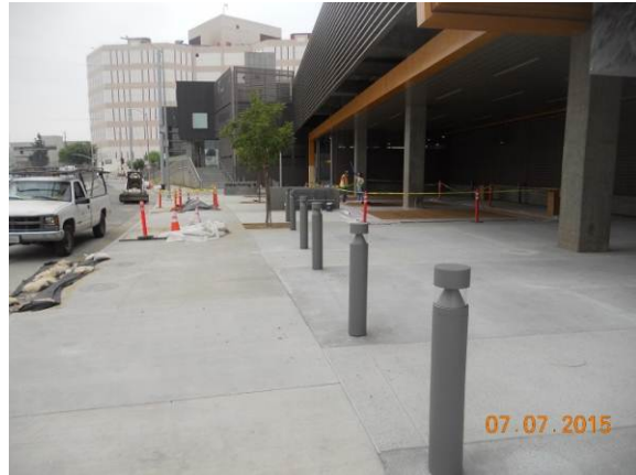
Striping and Landscaping work in progress at Div 13 West Side .
