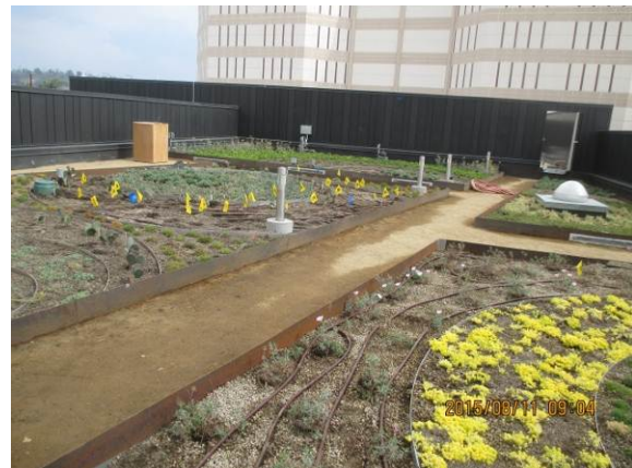
Vegetated Garden Roof Planting in progress.
