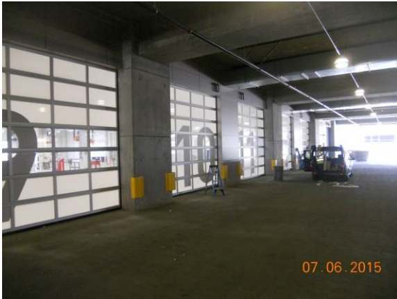
Signage on Maintenance Gates installation in progress.
