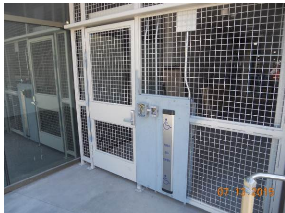
Accessibility equipment installation for DA in progress at Bldg A L1.
