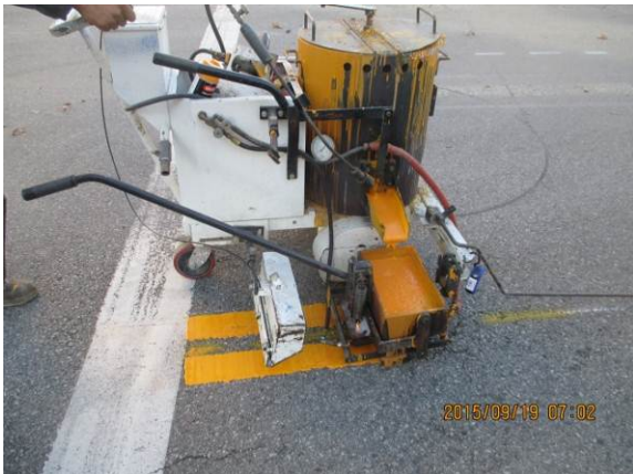
Vignes Street Striping commenced. Work completed same day.
