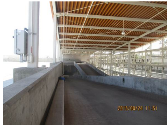
Cleaning completed at Parking Garage Ramps at Upper Level.
