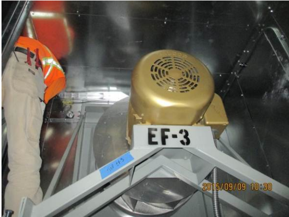
Exhaust Fan #3 installation in progress at Bldg. B Lower Level.
