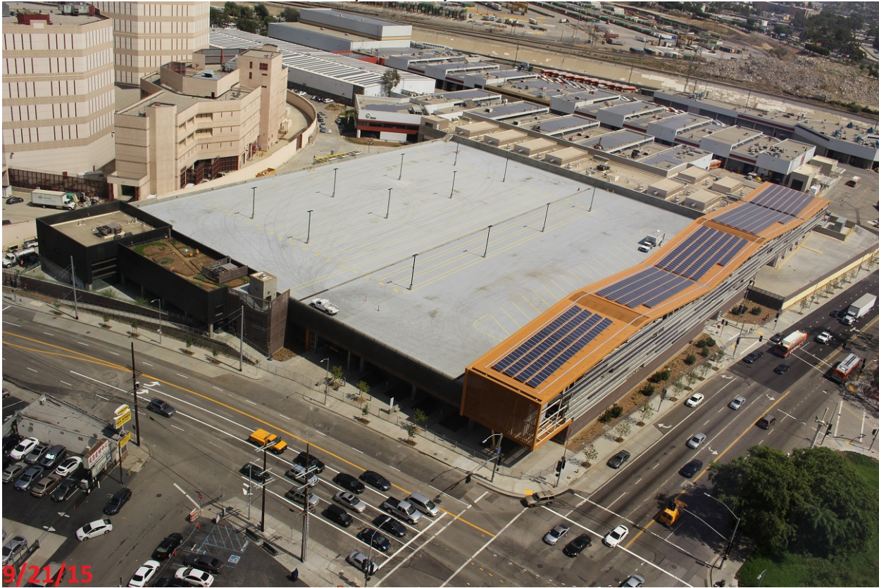
9/21/15 Transportation Building, Parking Garage and Maintenance Building in construction; at the bottom side Cesar Chavez Avenue and at the bottom left side Vignes Street with all lanes open.
