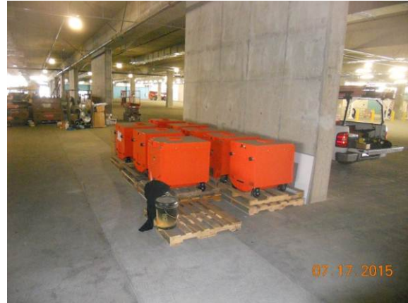
Fare Vaults on site at Bldg B Level 1, installation in progress.
