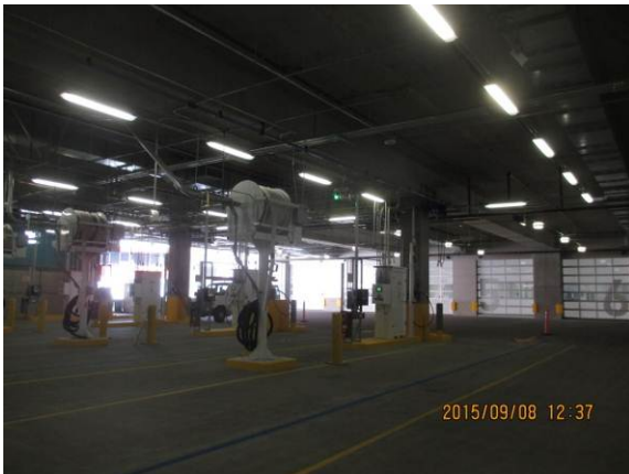
Striping and Painting completed at Fuel stations at Bldg. B Level 1.
