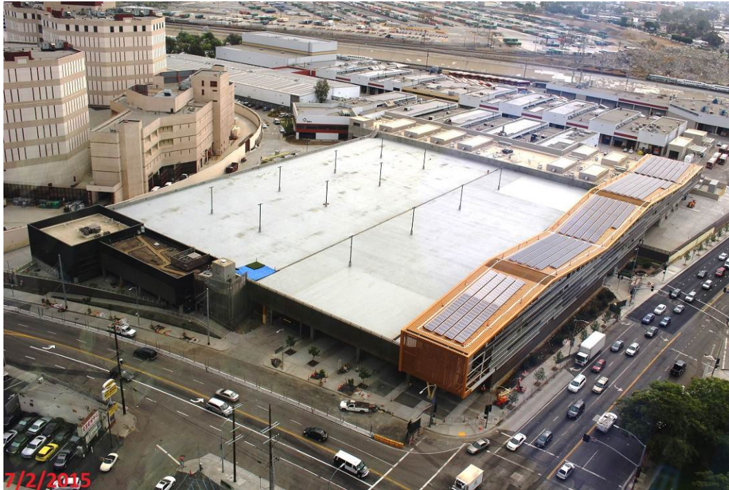
FLY OVER JOBSITE PHOTOGRAPH (7-2-2015)
