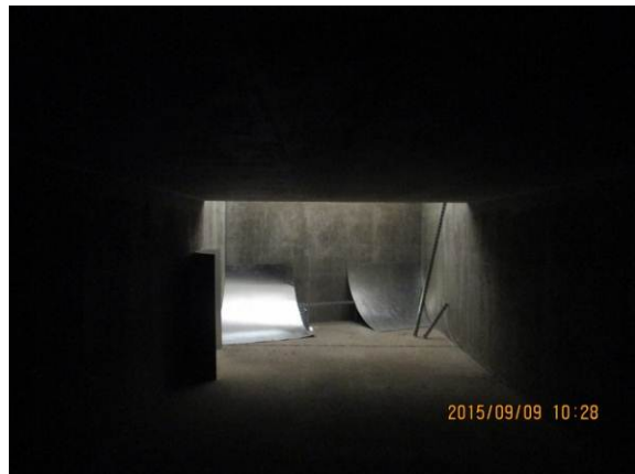
Flow Deflectors modification in progress at Parking Bldg. L.L.
