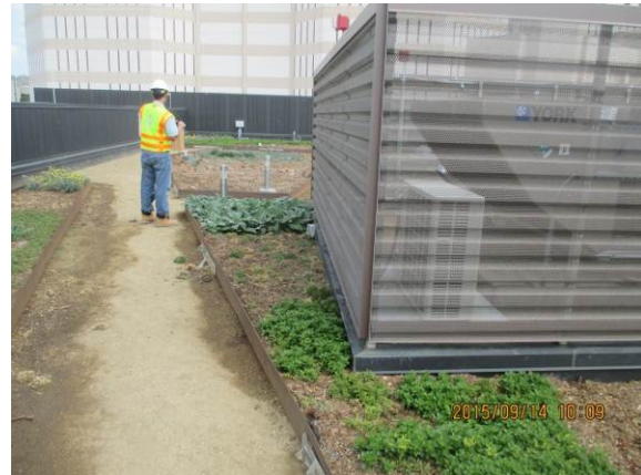
Vegetated Roof Garden Landscaping work completed.
