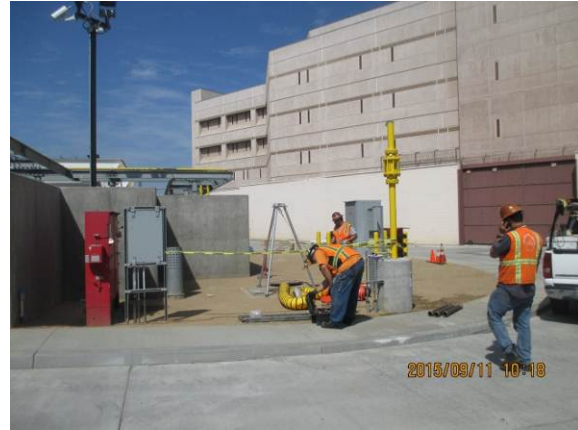
Plumbing and Cleaning work in progress at exterior CNG Facility.
