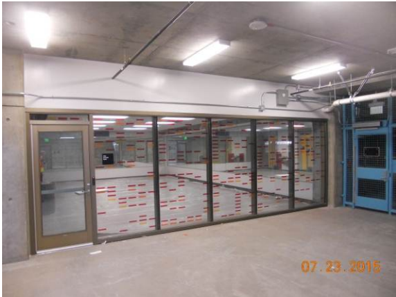
Glazing installation completed at Transportation Bldg. Lower Level.
