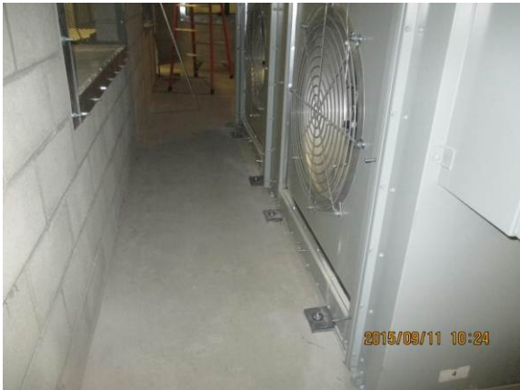
All EFs at redesign location, ready for installation & power .
