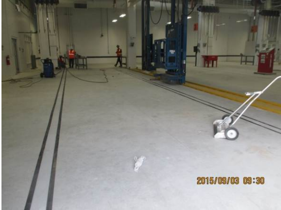
Prep & cleaning for striping work at North of Maintenance Bldg.
