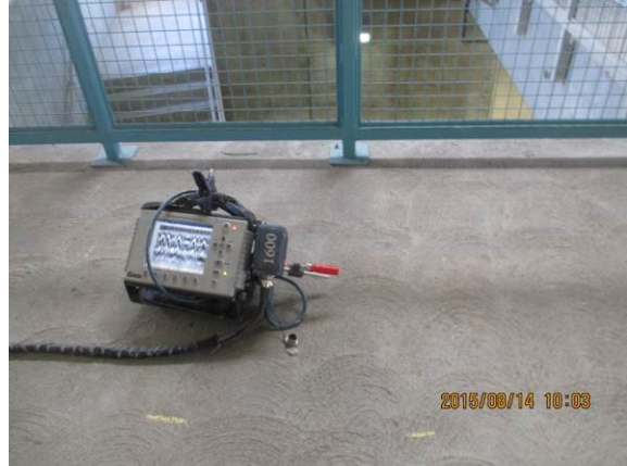
Ground Penetrating Radar (GPR) testing Parking Bldg Level 1.
