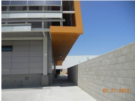
Lighting fixtures installation under East Wall Soffit completed.
