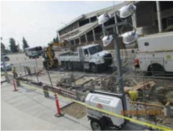
Existing sidewalk removal/ lanes construction at Cesar Chavez.
