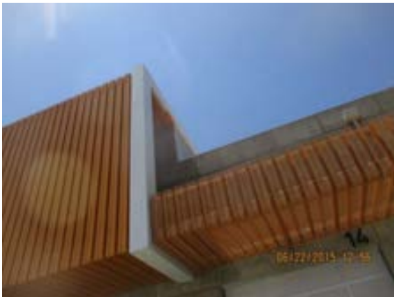
Perforated Steel Deck member installation completed at Bldg. C.
