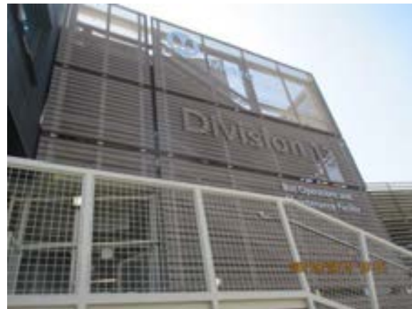
Metro Logo & Label Signs installation completed at Building A.
