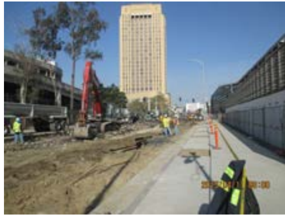
Street remodeling at Cesar Chavez Avenue.
