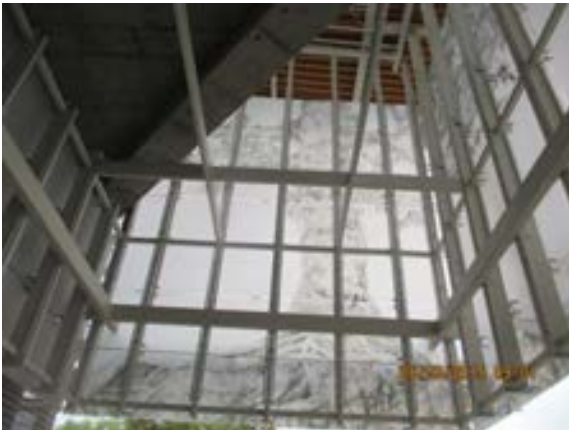
Artwork Panels installation completed at SW Corner.
