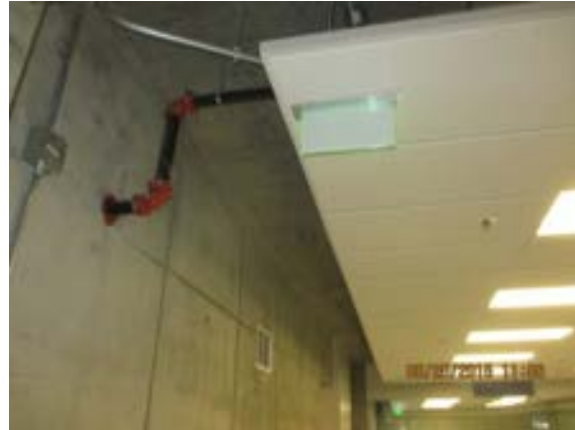
Signs & lighting fixtures changes done at Level 1 Building A.
