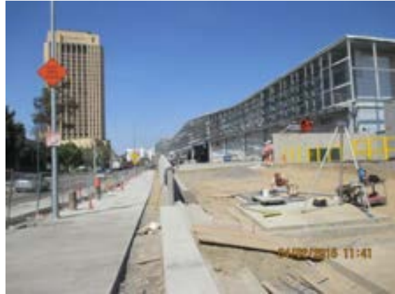
Utility Yard Water Jellyfish Tank and CMU preparation.
