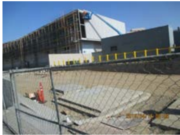
Steel deck installation in progress at Maintenance Bldg.
