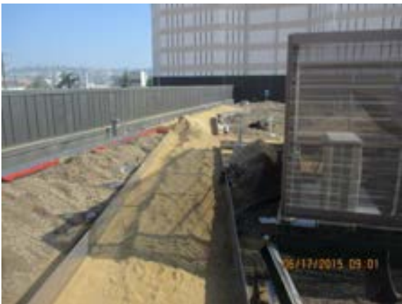
Earthwork & dirt application on vegetated roof at Building A.
