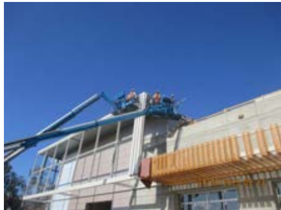
Work in progress at end of ribbon roof at Maintenance Bldg.
