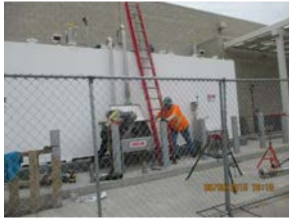
AST Hydraulics work in progress at Non-Revenue Fuel Area.
