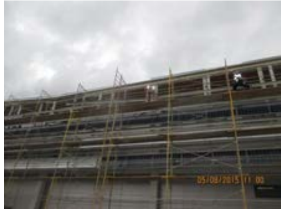
PV Panels installation in progress at south façade maintenance.
