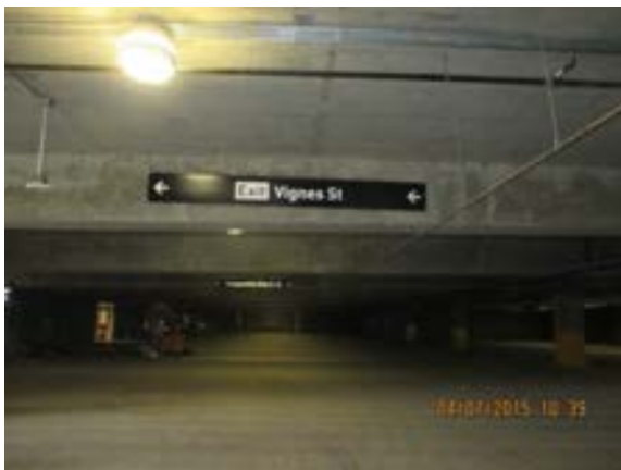
Signs installation completed at Lower Level Parking Garage
