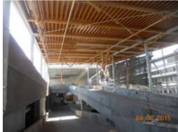
Ribbon roof painting & protection coat application in progress.
