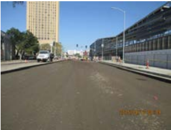
Cesar Chavez Ave second day of remodeling work.
