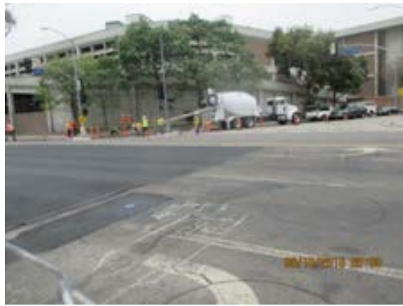
Southeast corner of Lyon St. final pouring in progress.
