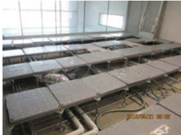
Clean up at raised up floor at 2 nd Level Transportation Building.
