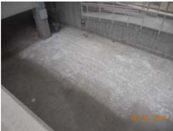
Grinding work at Lower Level Parking Garage in progress. .
