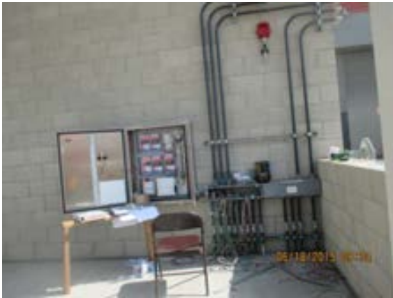
Electrical Components installation on Non-Rev Fuel Area.
