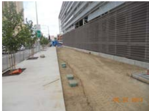
Street trees planting at south façade of Parking Garage Building.
