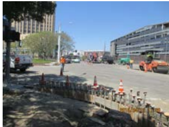
Sidewalk ramps construction & asphalt application at Cesar Chavez.
