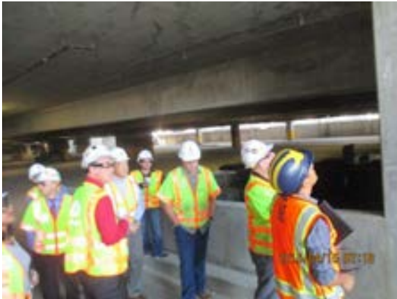
Metro PM & Structural Engineer at Project site view.
