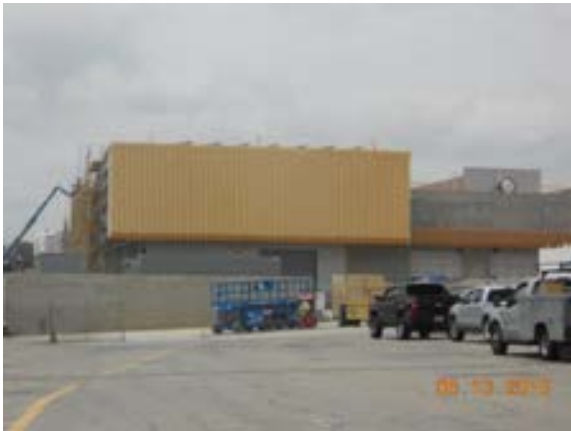
Steel deck vertical members installation in progress at Bldg. C.
