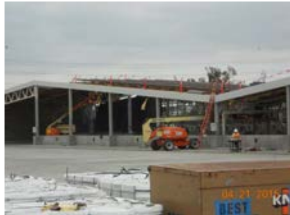
Installation of solar panels in progress on ribbon roof.
