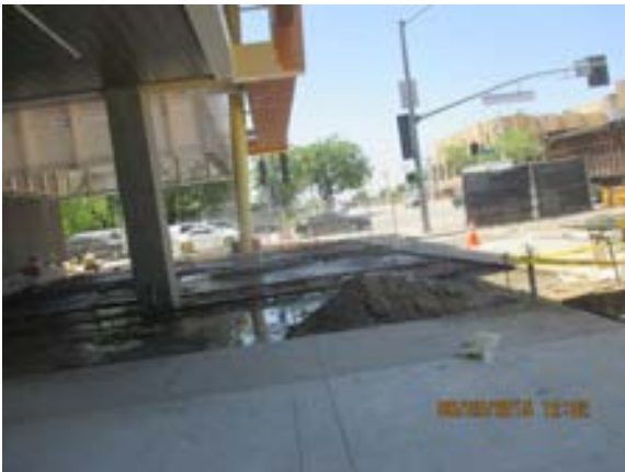
Preparation for Concrete pouring below Parking Garage Soffit.
