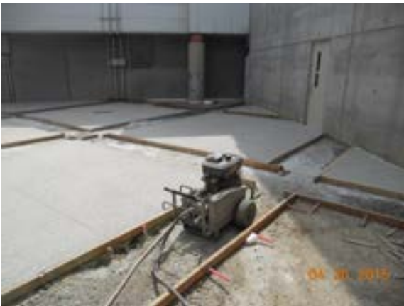
Concrete slab pouring between Bldg. 1 & Maintenance Bldg.
