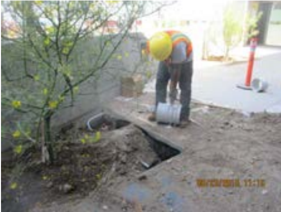
Landscaping work in progress at 1 st Level Transportation Building.
