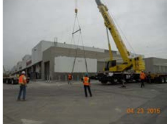
Installation of above Storage Tank at Chassis/Wash Area.
