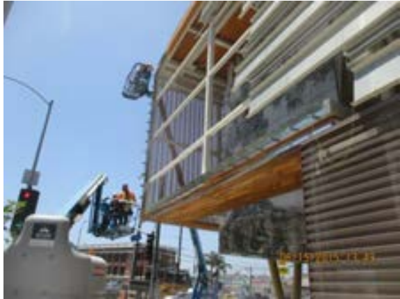
Perforated vertical/horizontal metal decks installed at SW Corner.
