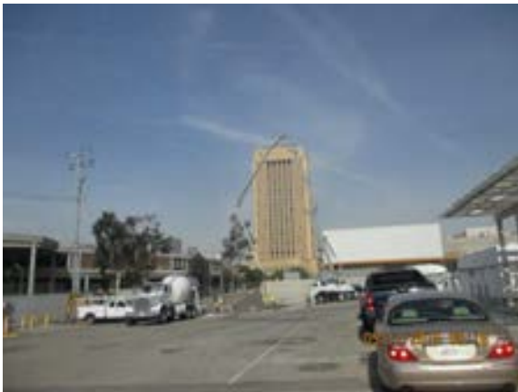
Concrete pouring & finishing at Utility Yard Area.
