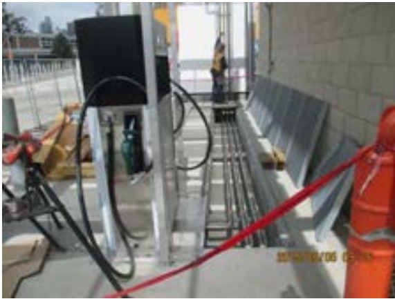
Mechanical/Plumbing components installation at Non-Rev Fuel Area.
