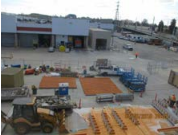
Steel deck on-site painting at Maintenance Bldg.
