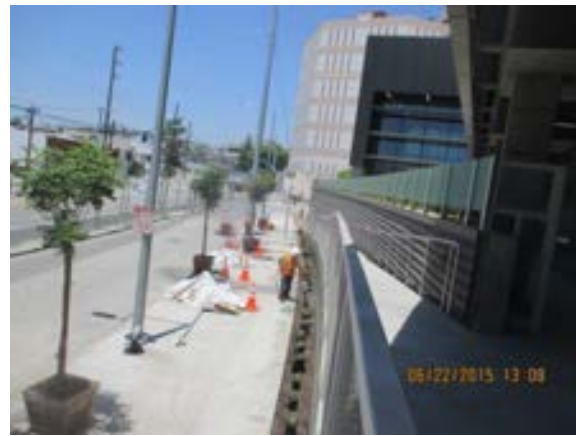
Irrigation & landscaping plants ready for planting at Building A.
