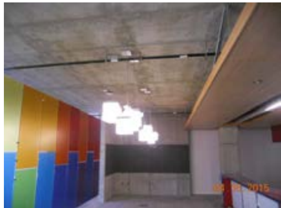
Lighting fixtures installation at Level 1 Transportation Building.
