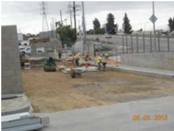
Concrete pouring preparation at Utility Yard Area.
