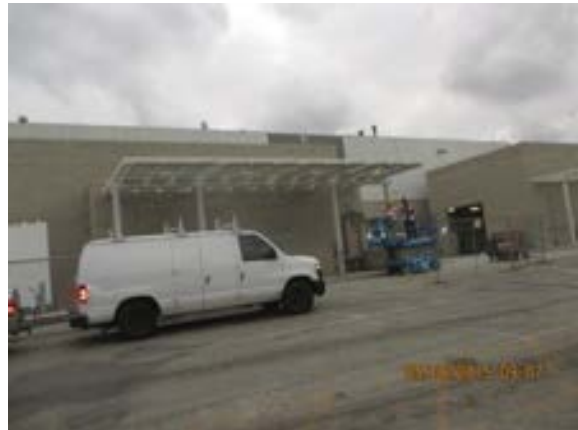
Perforated metal ceiling welding at Non-Revenue Area.
