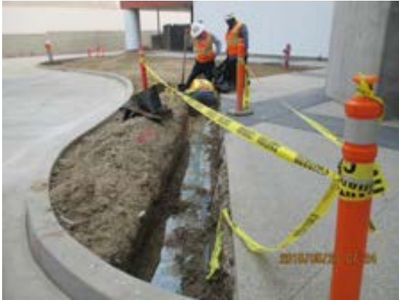
Landscaping work and clean up at Maintenance Building.
