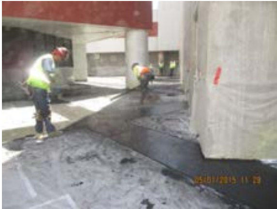
Concrete slab pouring finished between Bldg. 1 & Bldg. C.
