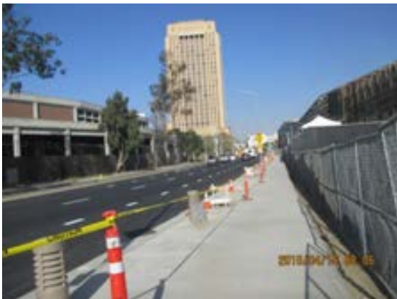
First coat of asphalt application at Cesar Chavez.
