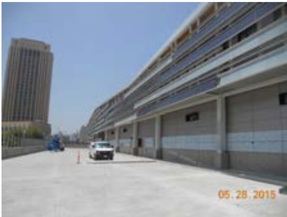
PV Panel Finish Bldg. A Level 1.
