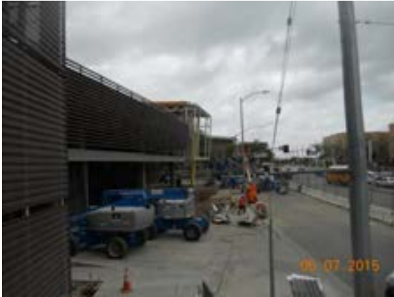
Artwork installation in progress at SW Corner along Vignes St.
