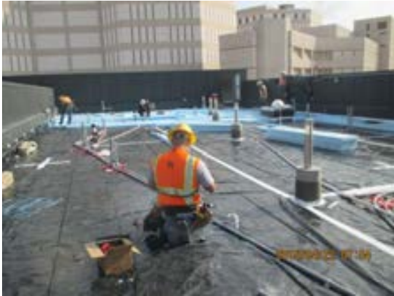
Styrofoam Insolation installation at Vegetated Roof at Bldg. A
