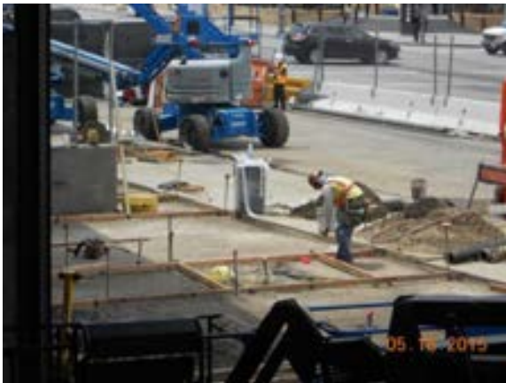
Earthwork and prep for concrete pouring at Vignes St. sidewalk.
