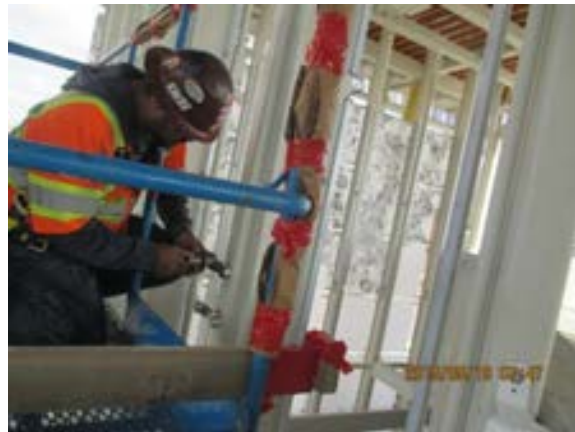
Artwork panels and electrical work installation at SW Corner.
