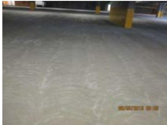
Grinding work at lower level Parking Garage completed.
