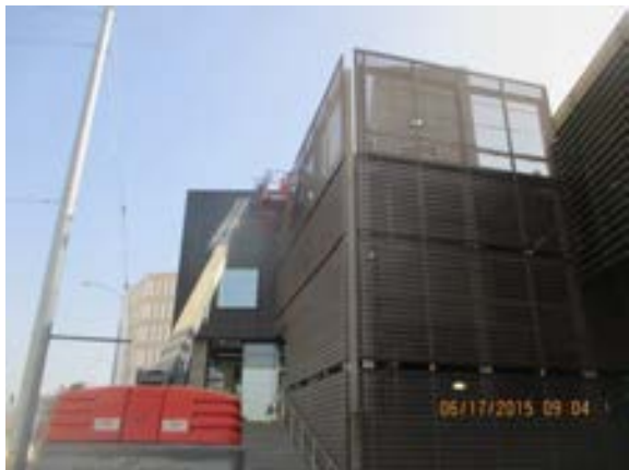
Metro Logo installation in progress at Transportation Building.
