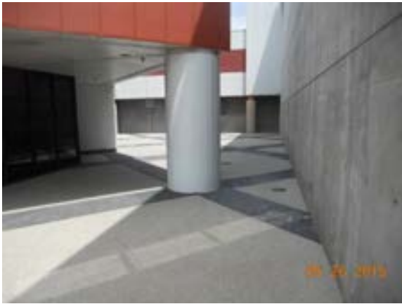
Concrete slab completed between Bldg. 1 & Maintenance Bldg.
