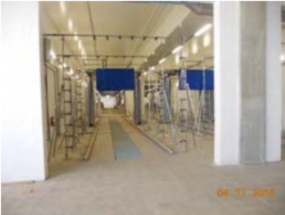
Bus wash work completed at Maintenance Building.
