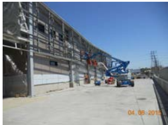
Final stage preparation for PV panels at south façade.
