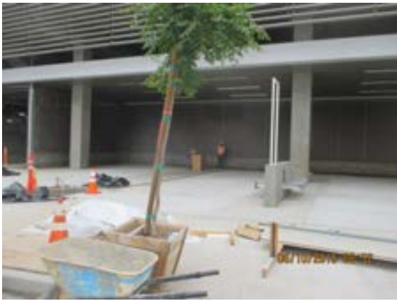
Street trees ready for landscaping/planting work.
