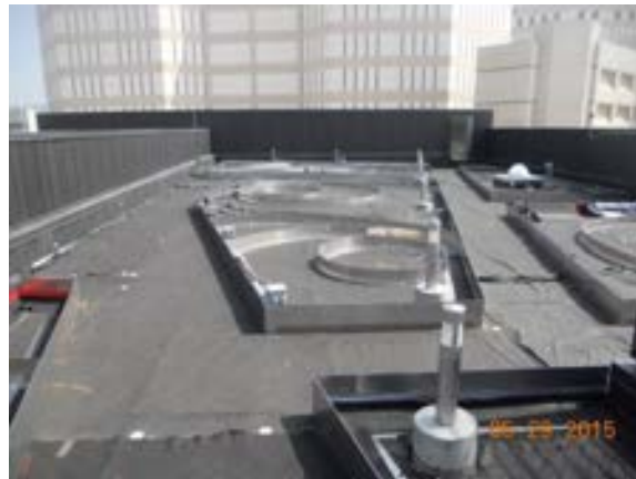
Vegetated roof plumbing components installation at Bldg. A.
