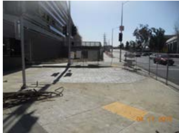
Concrete slab completed at Lyon Street driveway.
