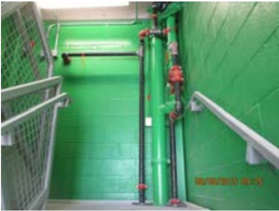
Painting work completed at stairs in Maintenance Building.
