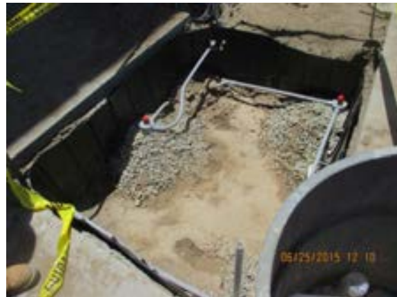
Electrical work in progress at Vignes St. driveway.
