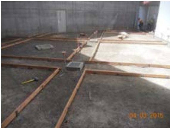
Concrete slab preparation between Bldg. 1 and 13 Bldg. C.
