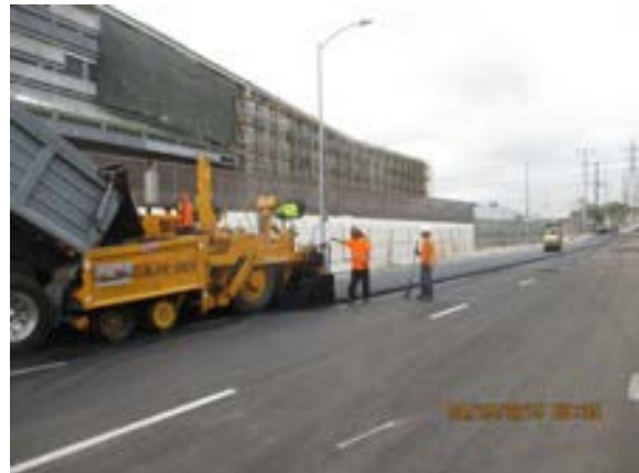
Application of final coat of asphalt at Cesar Chavez Ave.
