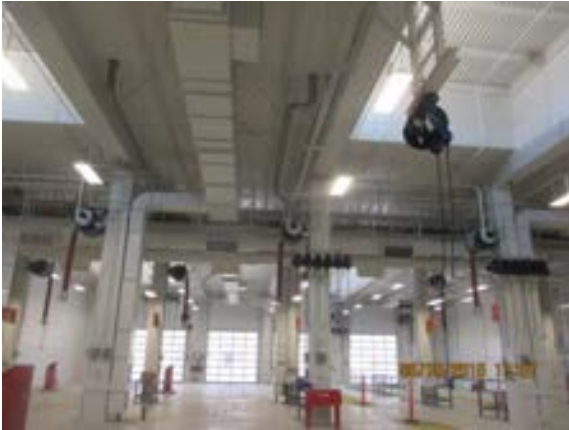
Work of Area 8 of Maintenance Building completed.
