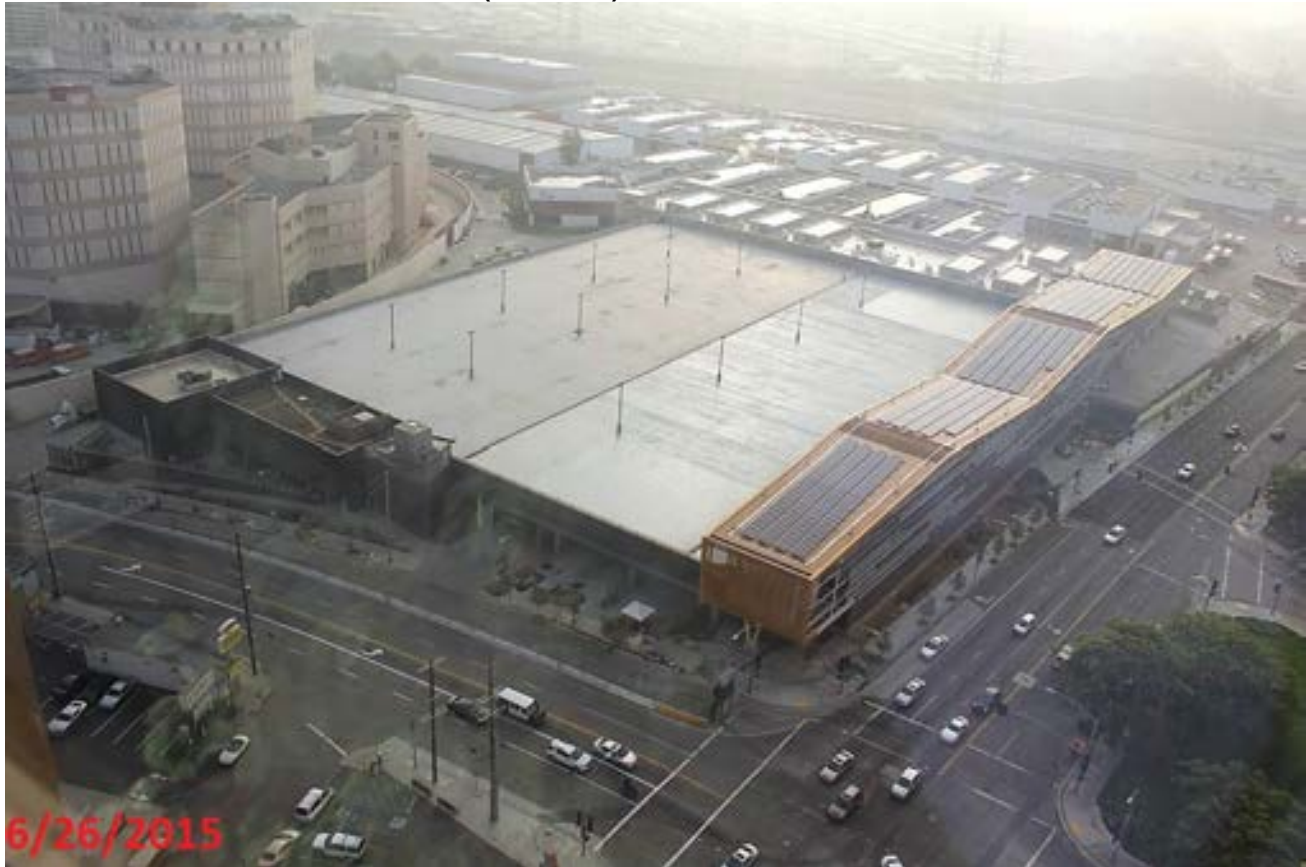
Transportation Building, Parking Garage and Maintenance Building in construction; at the bottom side Cesar Chavez Avenue and at the left side Vignes Street.
