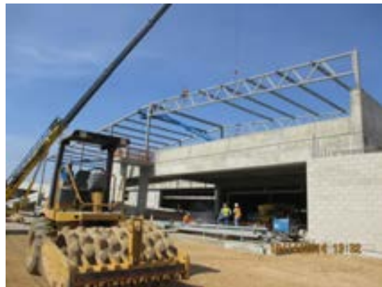
Erection of horizontal roof trusses at Parking Garage south.
