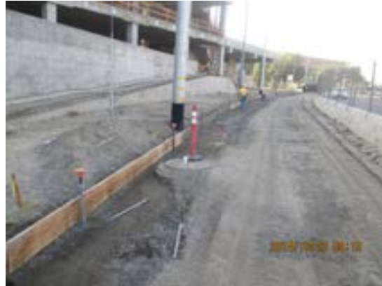
Installation of forms for street curbs and gutters at Vignes St.
