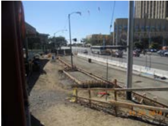
Form and rebar reinforcement of gutter and curbs at Vignes St.
