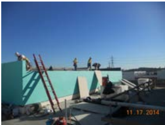
Installation of roof membrane at the Clerestory at roof level.
