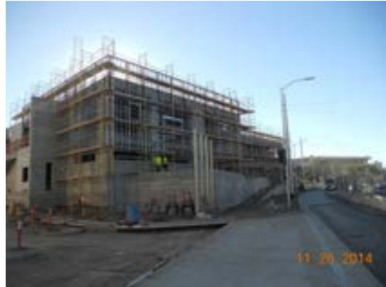
Exterior metal framing installation in progress at Transp. Bldg.
