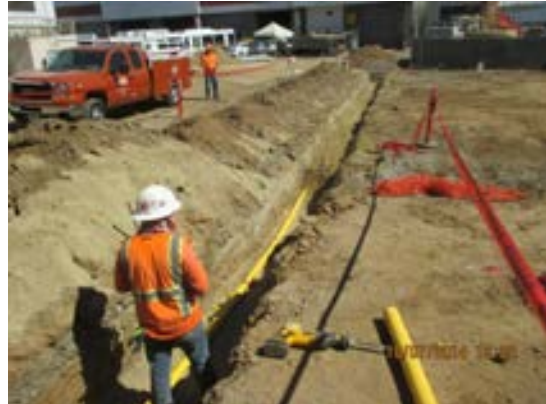
Installation of U/G gas pipe at east side of Maintenance Bldg.
