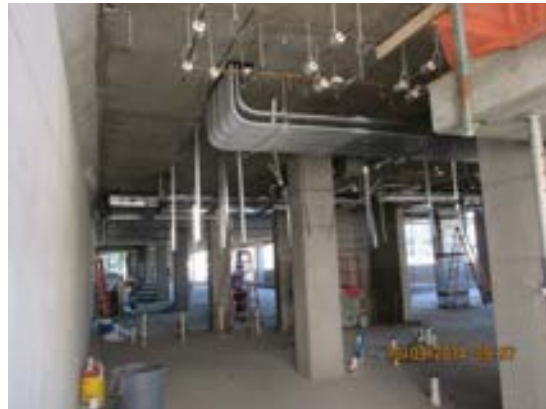
O/H elect. conduit installation at Transportation Building.
