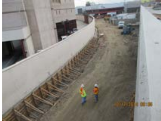
Retaining wall forms and rebar at Metro Driveway.
