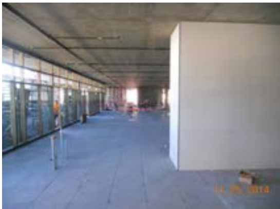
Placement of raised flooring panels at Transp. Bldg. Level 1.
