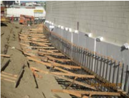
Form and rebar reinforcement of the retaining wall Metro Dr.
