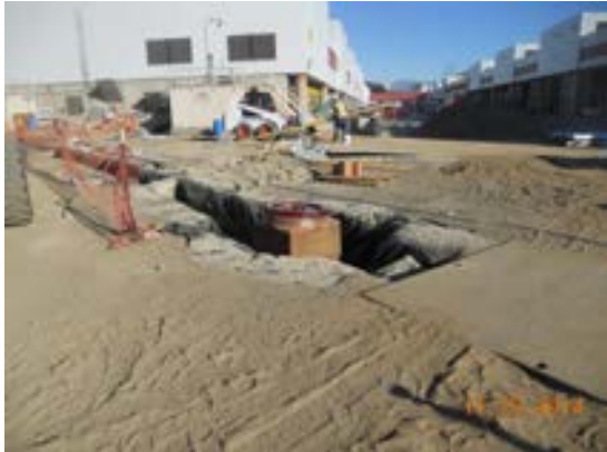
Installation of sump for the Genset fuel line to Chassis Wash.
