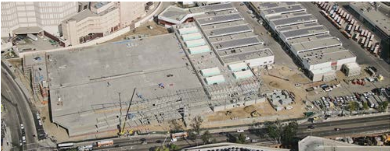
Transportation Building, Parking Garage and Maintenance Building in construction; at the bottom side Cesar Chavez Avenue and at the left side Vignes Street.
