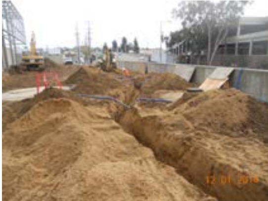
Excavation for storm water lines to the Water Tank #1.
