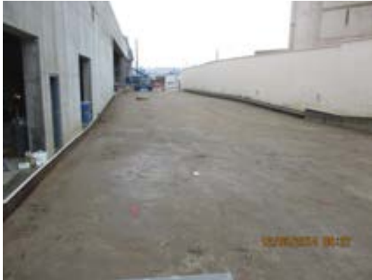
Finish compaction at Metro Driveway.
