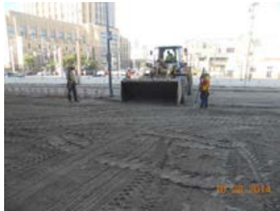
Prep work for the approach to the ramp at Vignes St.
