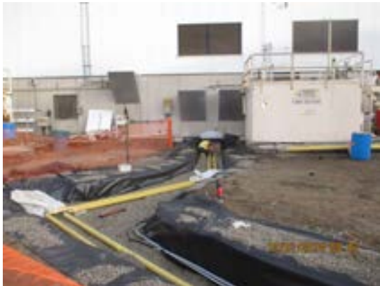
Placement of Genset fuel lines to the Chassis Wash Area.
