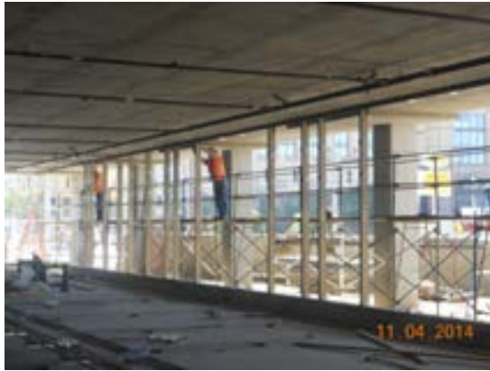
Installation of window metal framing at Transportation Bldg.
