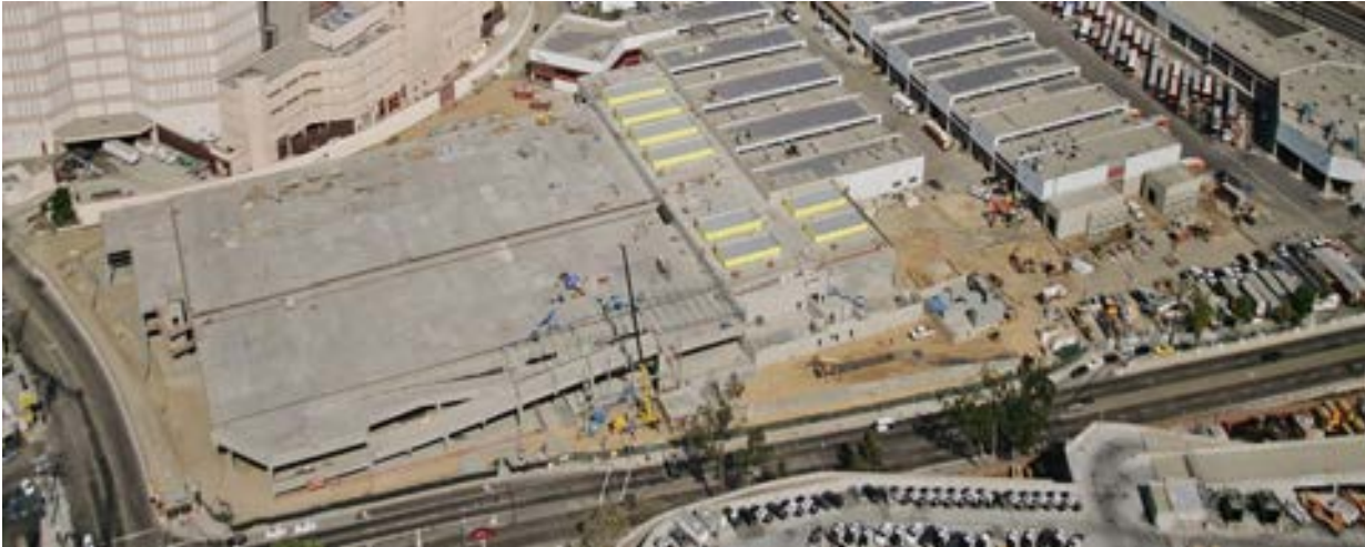
Transportation Building, Parking Garage and Maintenance Building in construction; at the bottom side Cesar Chavez Avenue and at the left side Vignes Street.
