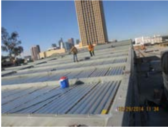
Installation of corrugated steel roof deck in progress.
