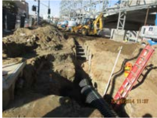
Installation of UG storm water lines at the Water Tank No. 1.
