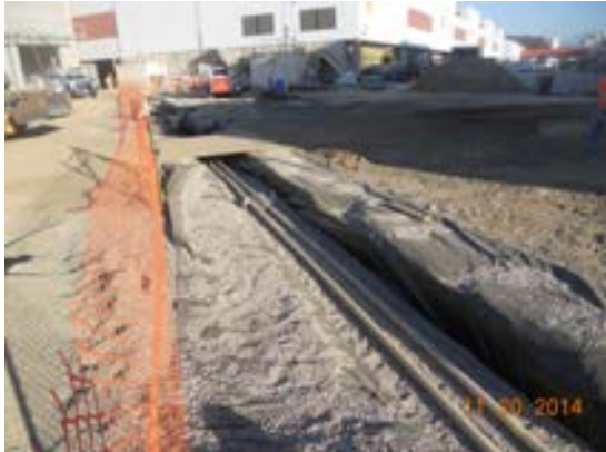
Placement of UG Genset fuel gas line at the Chassis Wash.
