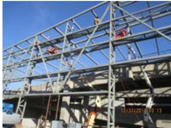
Installation of catwalk system at the roof deck in progress.
