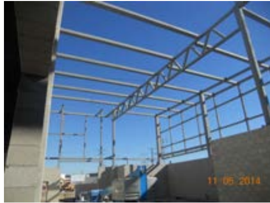
Erection trusses for the roof ribbon at Parking Garage.
