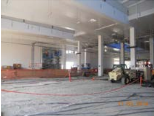
Applied prime and first coat paint at Maintenance Building.
