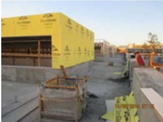
Exterior sheathing board installation at Clerestory at roof deck.
