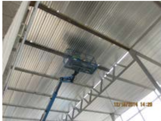
Installation of corrugated steel roof deck at Maint. Bldg.
