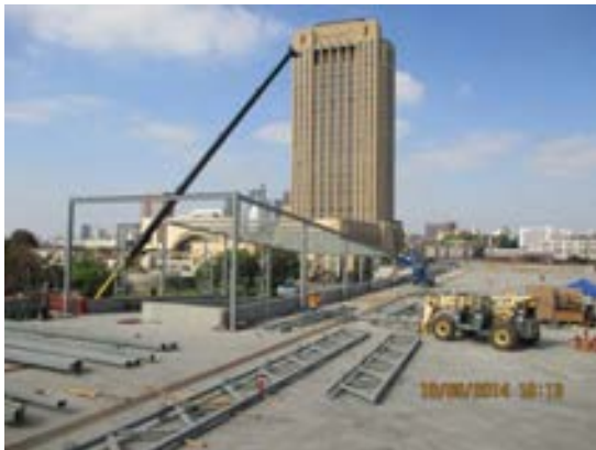
Installation of south elevation ribbon roof structural steel.
