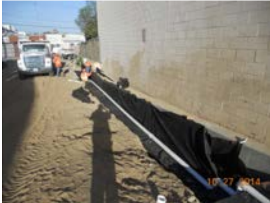
Water proofing along Metro Driveway retaining wall.
