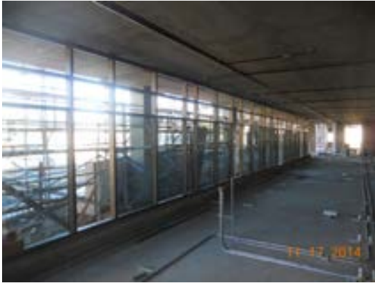
Installation of curtain wall at Transp. Building Level 1.
