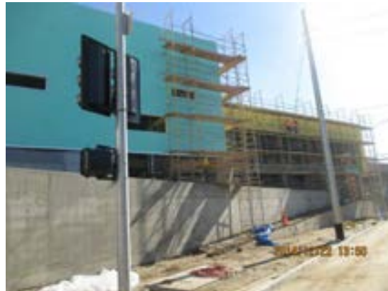
Installation of exterior sheathing at Transportation Building.
