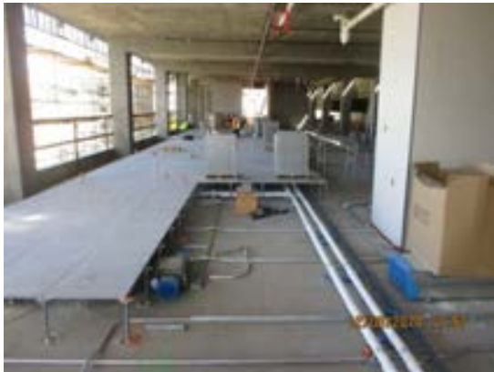
Installation of raised flooring in progress at Bldg. A Level 2.
