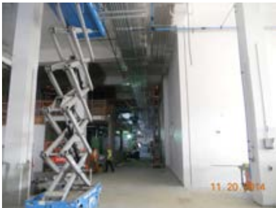
Installation of overhead MEP at Maintenance Bldg. Area 8.
