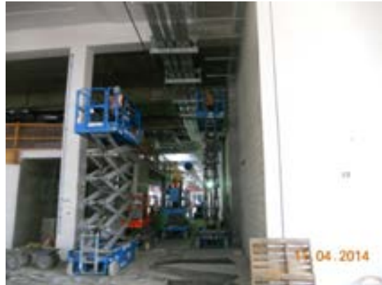
O/H Bus Duct installation at Maintenance Building.
