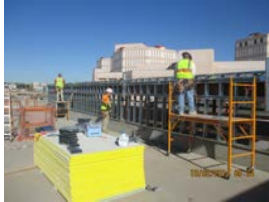
Installation of metal framing at roof level decks Areas 8, 9 & 10.
