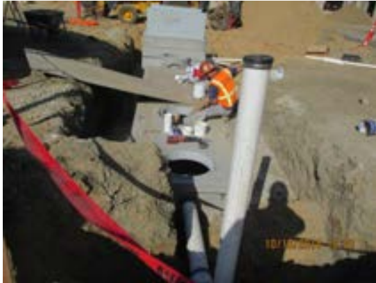
Installation of oil interceptors at east side of Maintenance Bldg.
