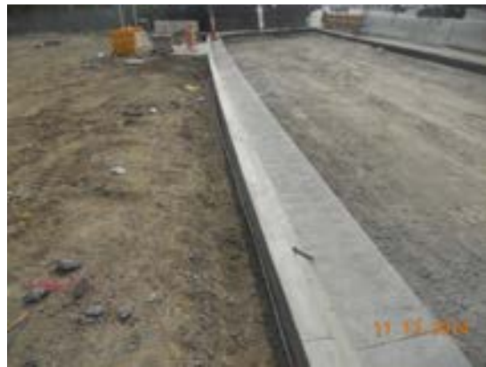
Concrete curb installed along Vignes St.
