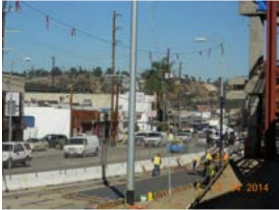
Concrete placement at bus pad on Vignes St.
