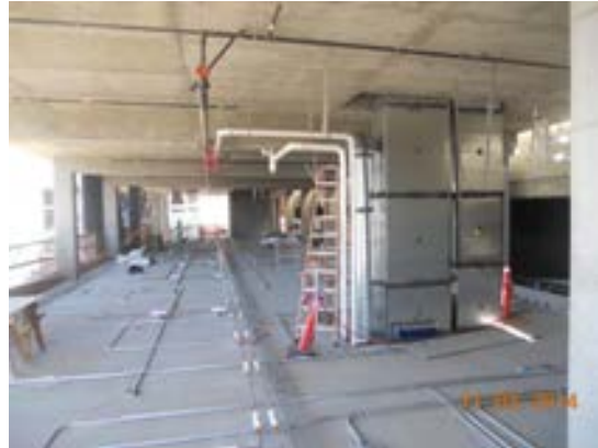
Installation of elec. conduits at Level1 Transportation Bldg.
