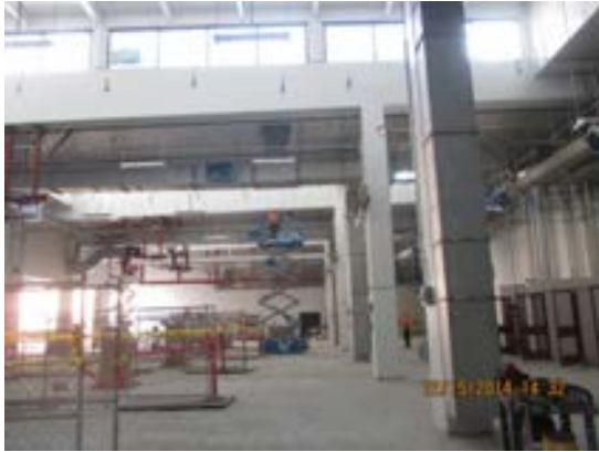
Overhead MEP installation in progress of Area 8.
