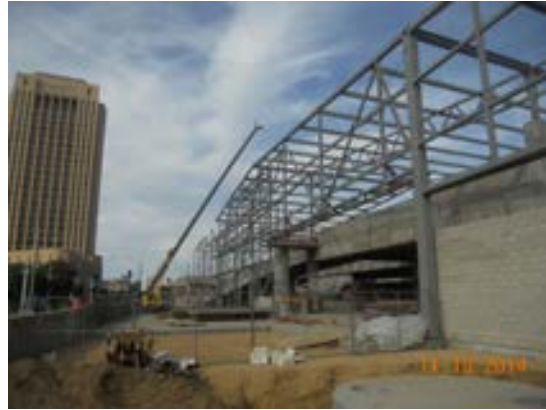
Erection of trusses for the roof ribbon at Parking Garage.
