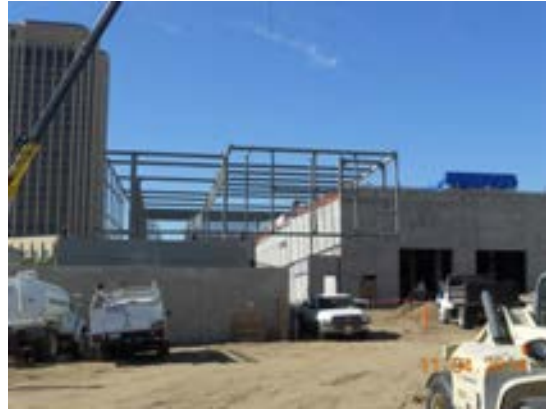
Installation of Roof Ribbon Systems at Maintenance Building.
