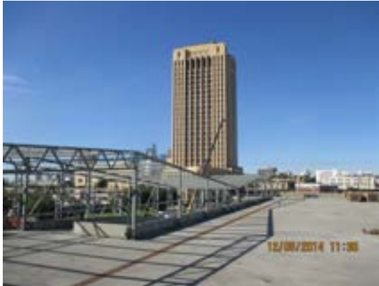
West view of steel roof ribbon system installation in progress.
