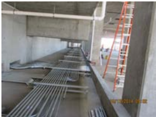
In progress electrical conduit installation Transp. Building.
