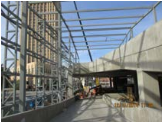
Installation of steel Roof Ribbon System in progress.
