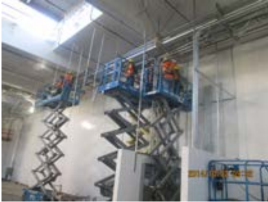
O/H electrical conduits installation Maintenance Building.
