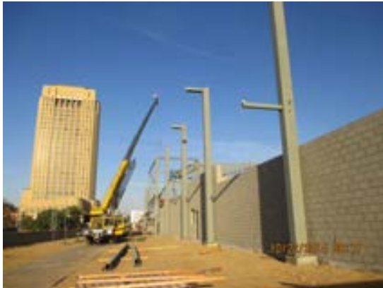
Erection of main roof members at the Maintenance Bldg.
