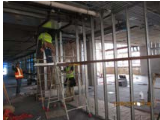
Installation of interior metal framing at Bldg. A Level 2.
