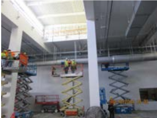
Installation of O/H HVAC exhaust duct at Maintenance Bldg.
