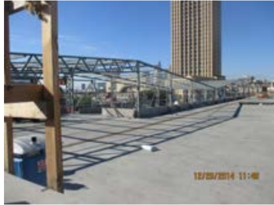
Installation of steel roof ribbon system in progress at Bldg. B.
