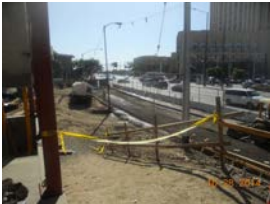
Placement of aggregate base at Vignes St.
