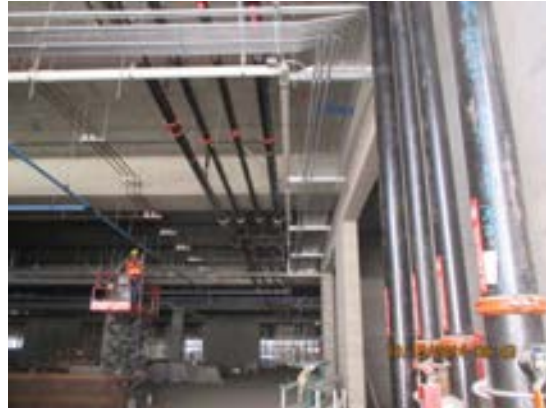
In progress O/H piping installation at Level 1 Parking Garage.
