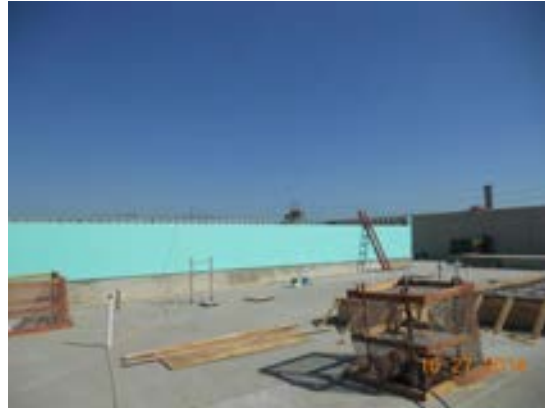
Applied liquid waterproofing at Clerestory at Building C.
