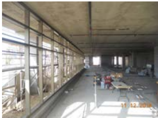
In progress installation of window framing at Trans. Building.
