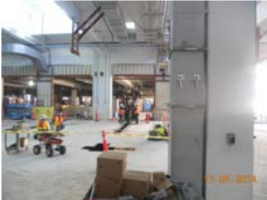
Interior view at Maintenance Building Level 1.
