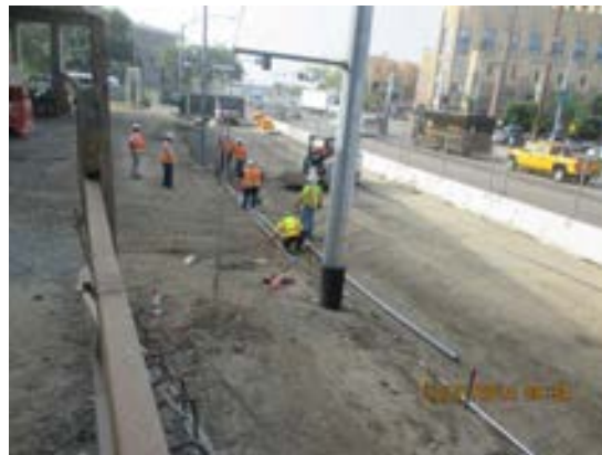
Installation of electrical conduit for light poles at Vignes St.
