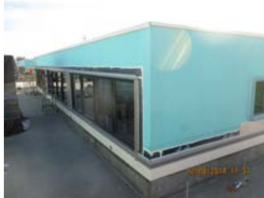
Installation of glazing at Clerestory at roof deck Bldg. B.
