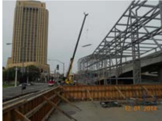
Erection of steel roof Ribbon Assembly System.
