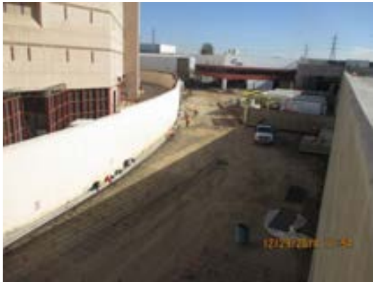
Installation of steel rebar basket in progress at Metro Drive.
