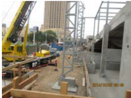
Erection of vertical trusses for the roof at Parking Garage.
