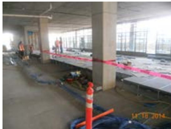
Installation of raised flooring panels at Level 1 Transp. Bldg.
