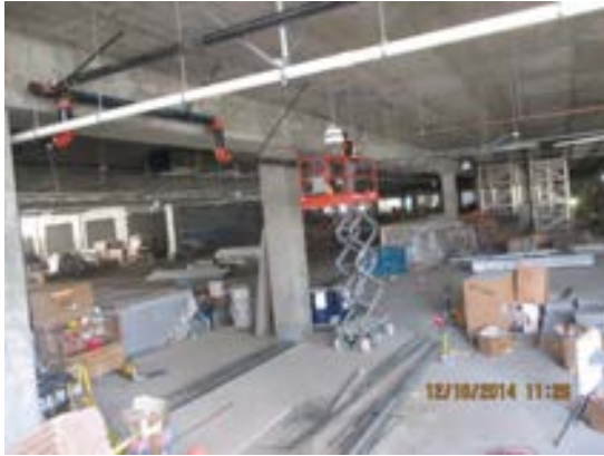
Installation of overhead light fixtures at Level1 Bldg. B.
