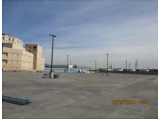
Light poles at the roof deck of Parking Garage.
