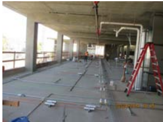
Installation of elec. conduits at Transportation Building.
