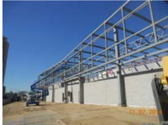
Side view of roof ribbon installation at the Parking Garage.
