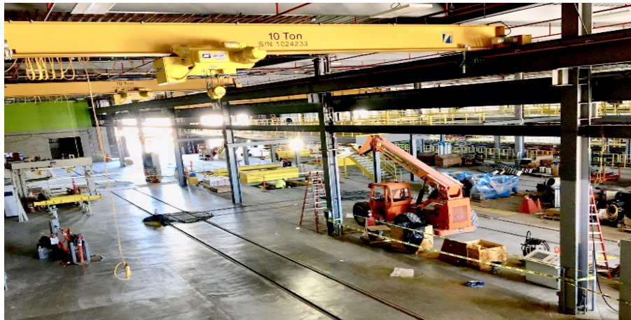
Southwestern Yard – maintenance area.
