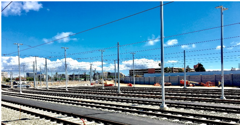
Southwestern Yard – storage tracks.
