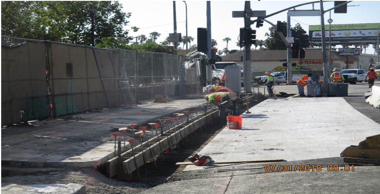
UG4/VERNON RESTORATION – Formwork for east curb and gutter between 43rd street and Vernon.
