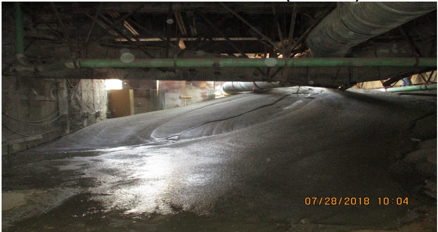
MARTIN LUTHER KING JR. STATION- Slurry backfill underneath utilities at the roof.
