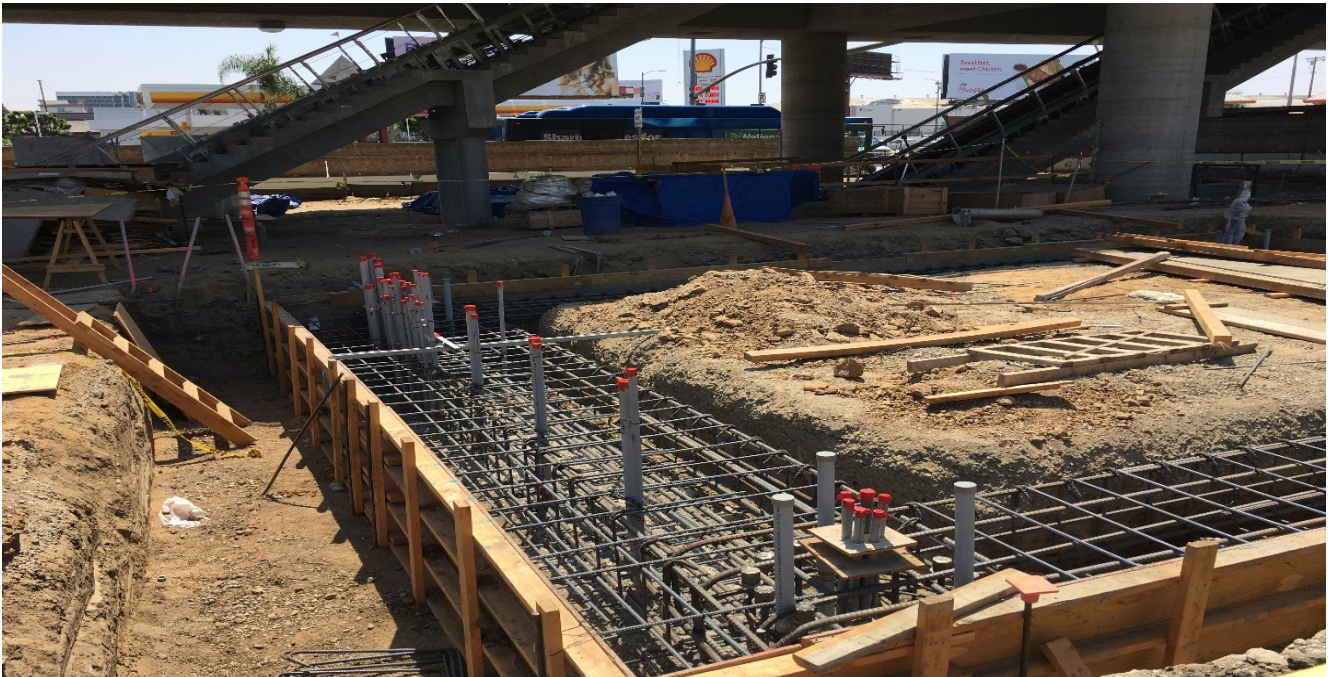
AVIATION/CENTURY STATION - All PVS Stubs have been raised above the pour line for the forms for the TVM's.
