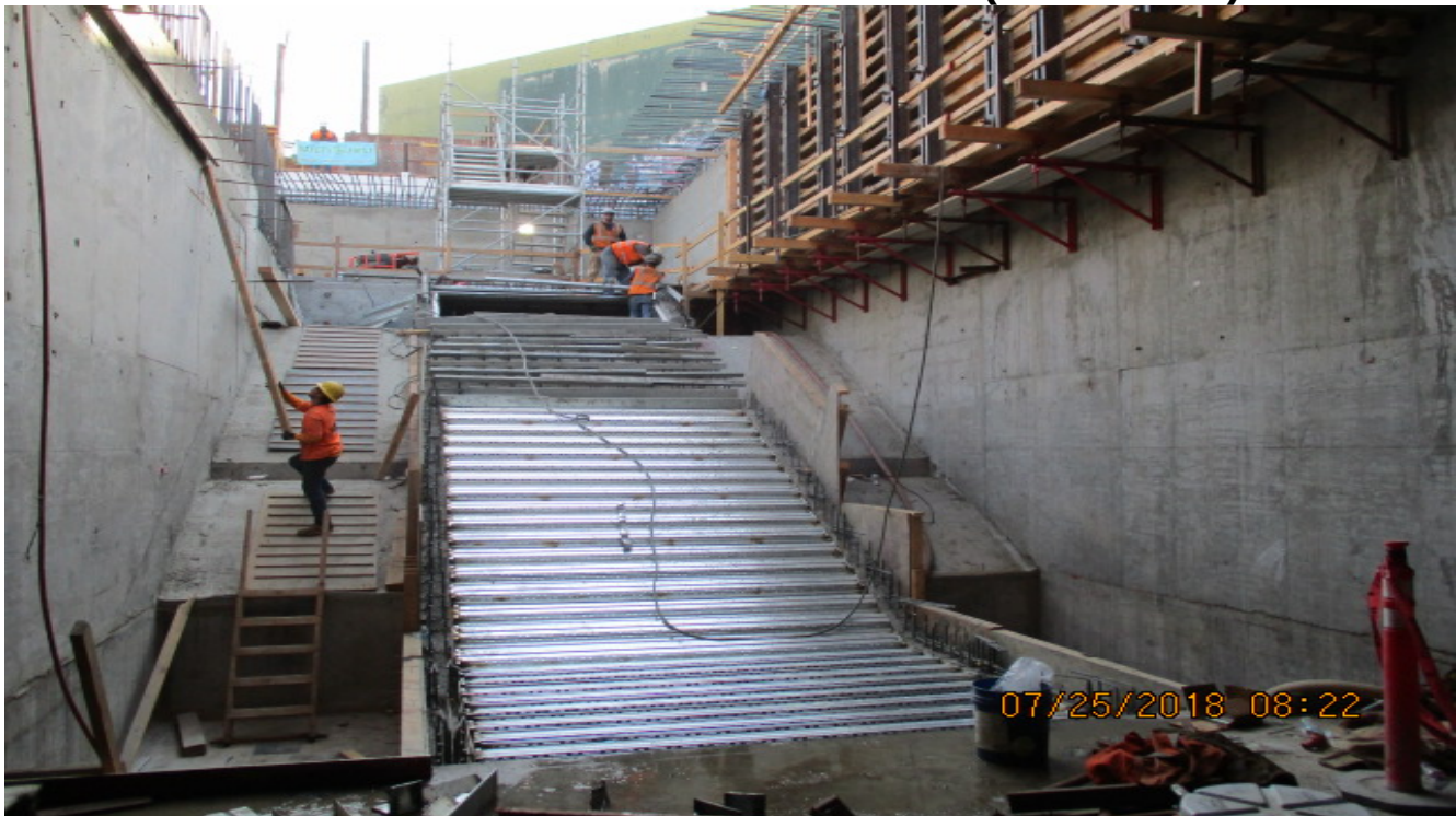
LEIMERT PARK STATION – Installation of anchors for the metal ceiling system above the platform.
