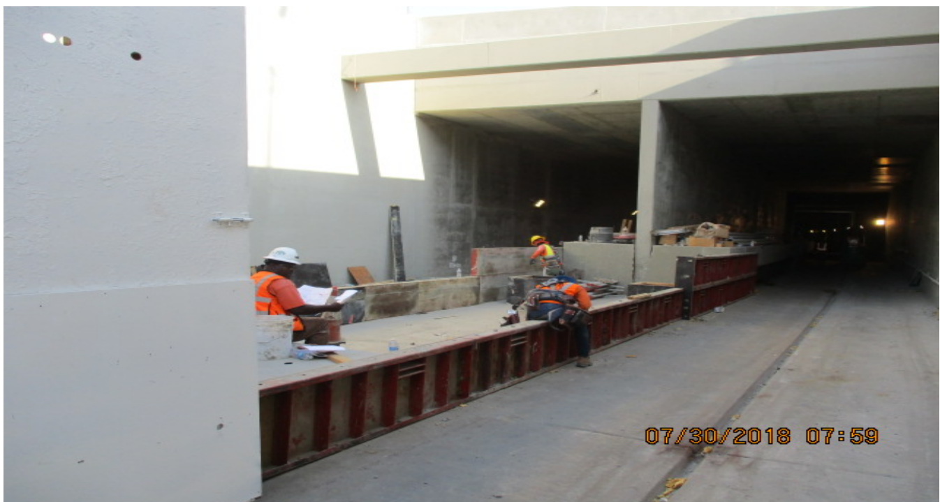
UG4 – Formwork for the remaining section of the emergency walkway at the south portal
