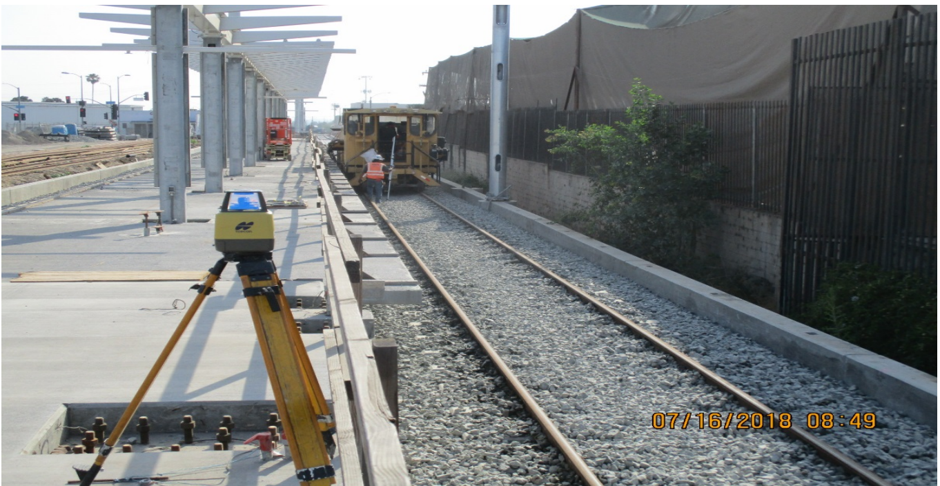
FAIRVIEW HEIGHTS STATION - Track 4 tamping and ballast regulating at the Fairview Heights Station.
