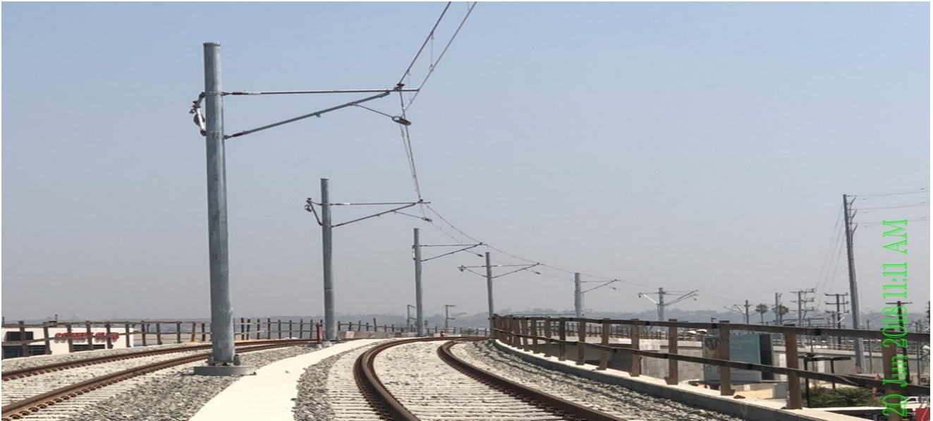
(AG-4) MANCHESTER BRIDGE – Crew installing messenger wire run WR #14.
