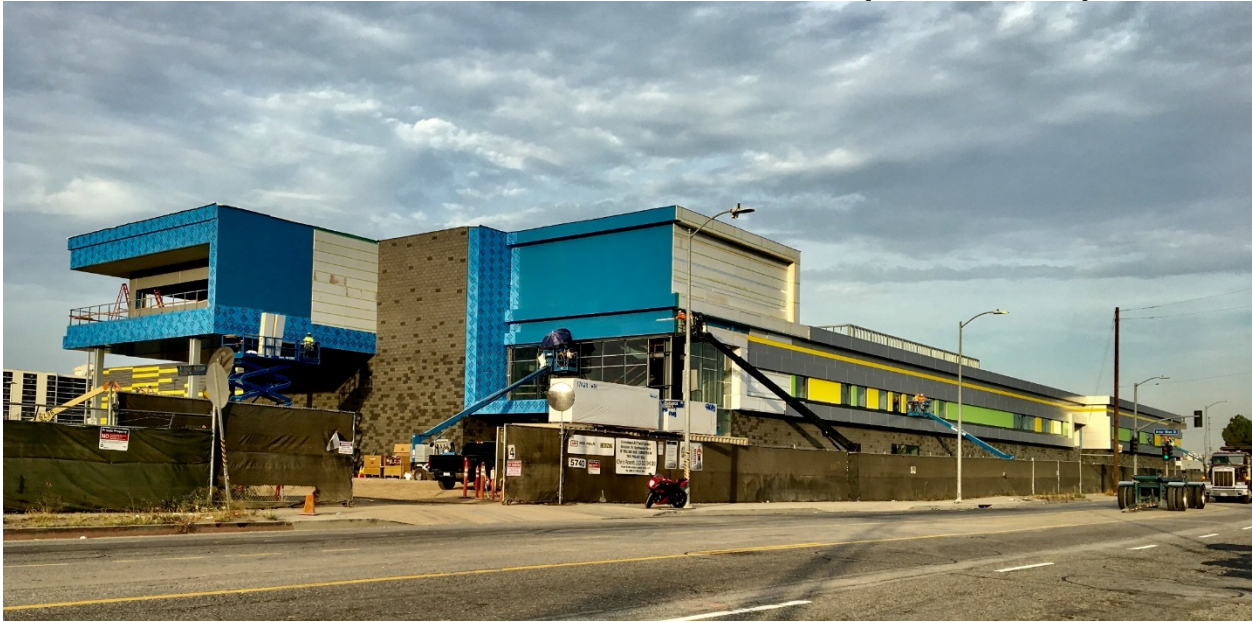
Main shop exterior finishes within the Southwestern Yard site looking southwest.
