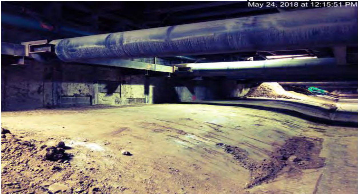
EXPOSITION/CRENSHAW STATION – backfill activities at the crossover roof (phase 4).
