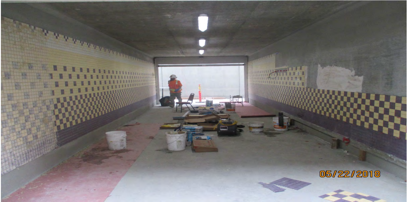
FCBC - setting tile for the walkway underpass.
