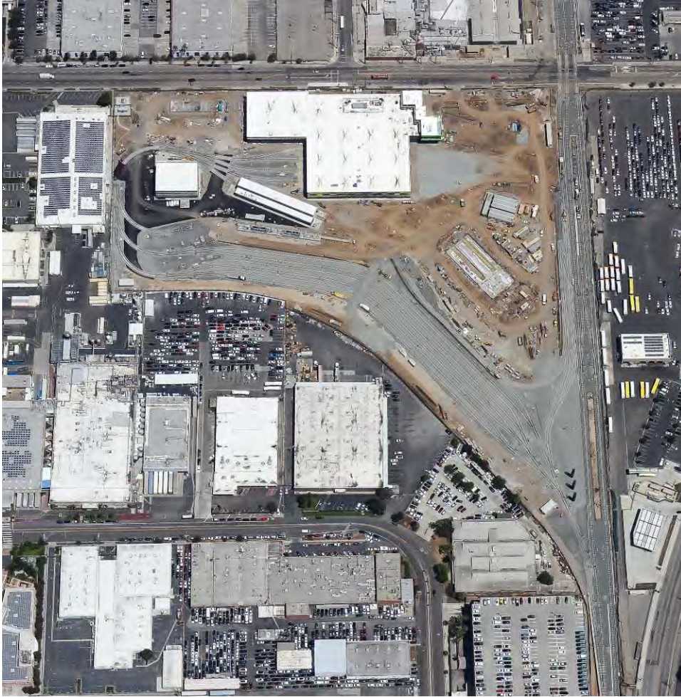
Aerial view of Southwestern Yard.
