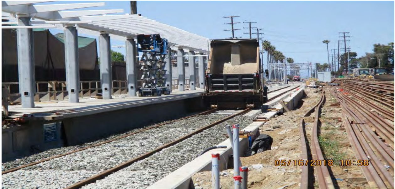
FAIRVIEW HEIGHTS STATION- top ballast rock spreading along southbound track.
