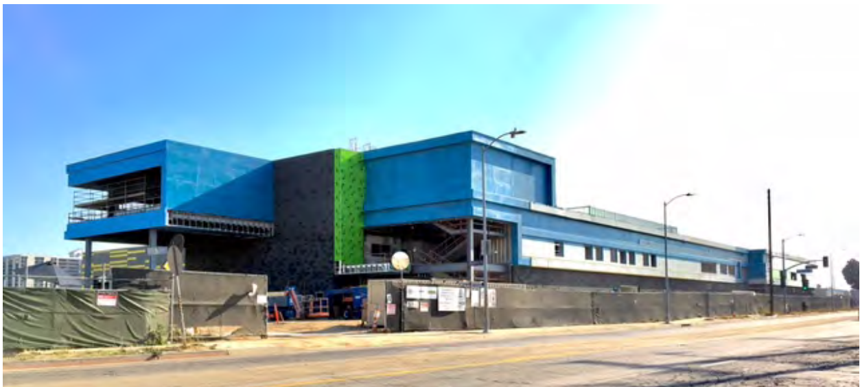
Main shop within the Southwestern Yard site.
