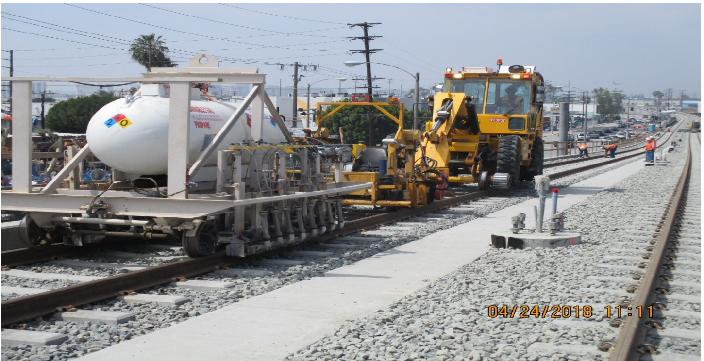
MSE 140L&R - Track 3 destressing and weld placement, & emergency walkway ballast placement.
