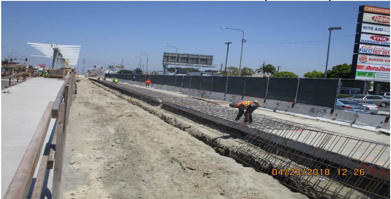
HYDE PARK STATION - Installation of rebar for ballast walls.
