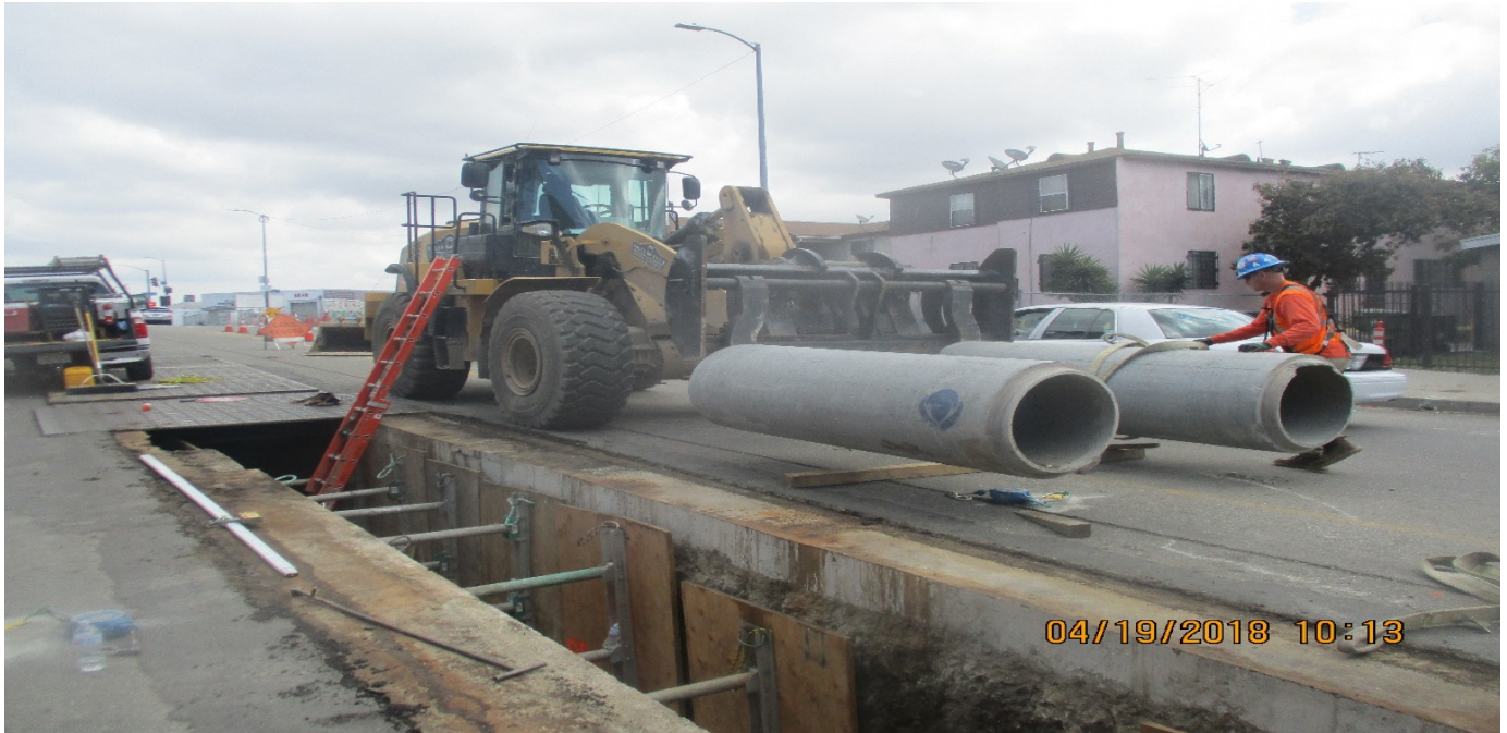
B1 GUIDEWAY - Placing 24 inch RCP SD on West St.
