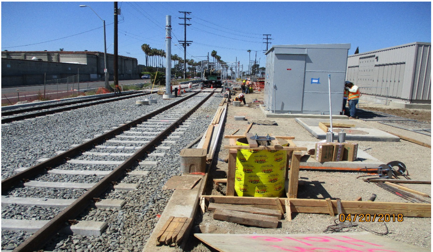
TPSS- TPSS 6- Foundation for site lighting.
