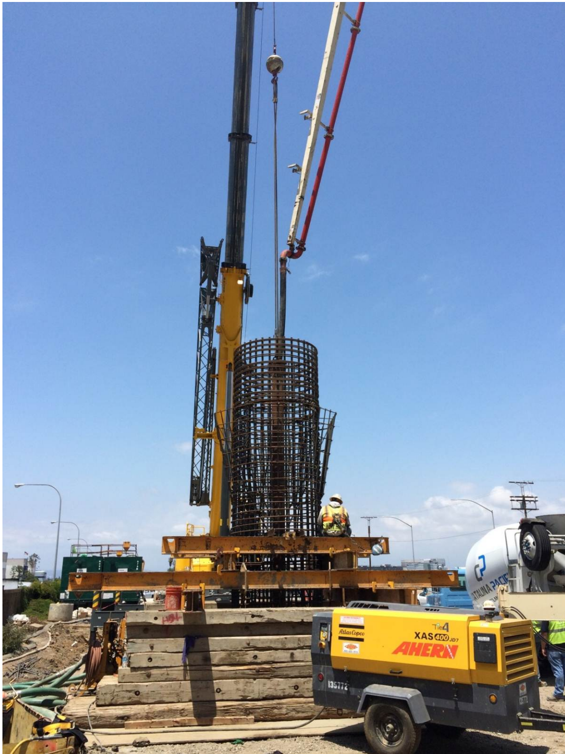
Concrete Placement for CIDH #5 (Bent 5).
