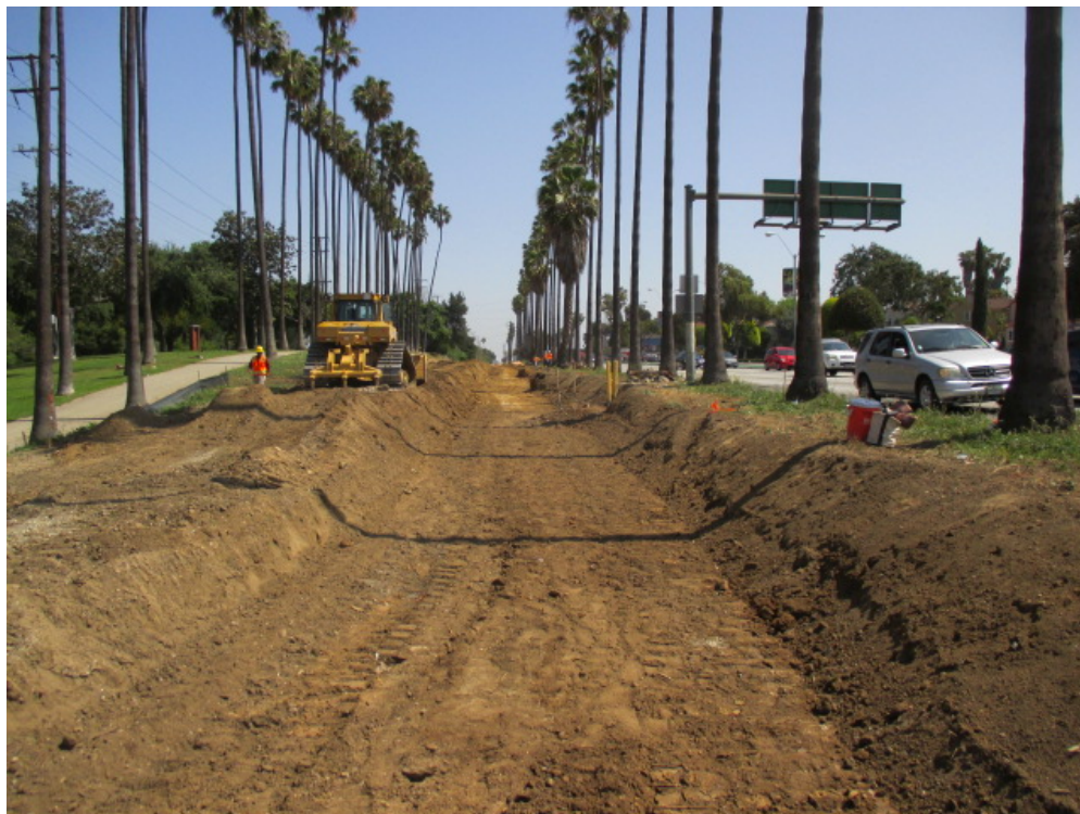
Florence Between Centinela and Redondo Clearing for Guideway Installation and Utility Investigation.
