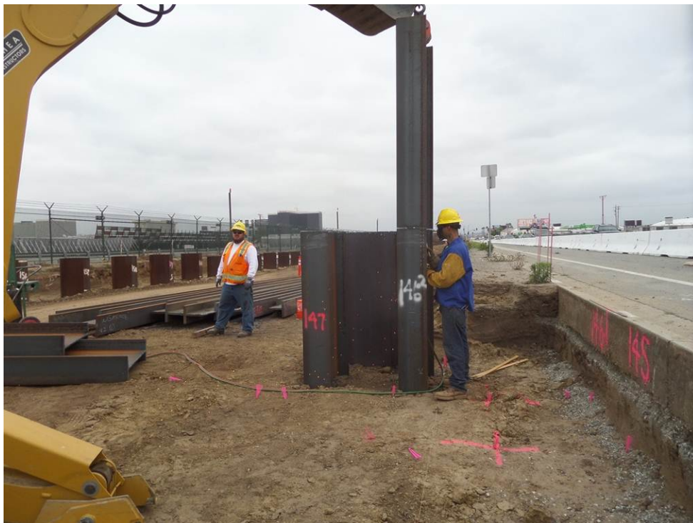
Topping SOE Piles at Emergency Stair Case 2.
