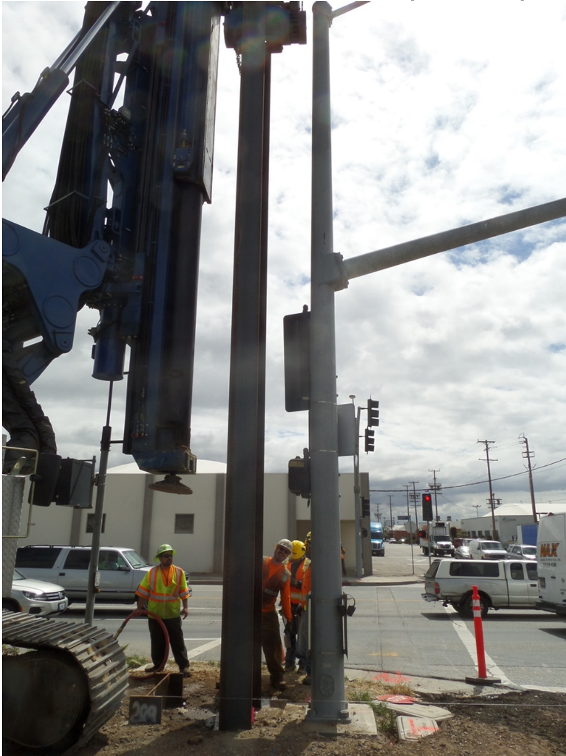
Installing SOE Pile 288.2 North of 104 th Street.
