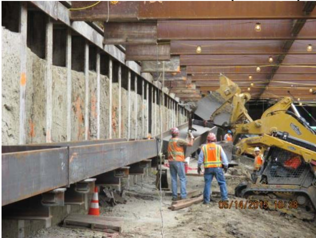
Installing West Walers at the MLK Station.
