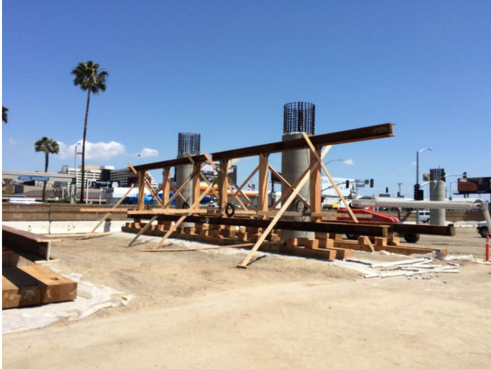
Aviation Century Underpass Falsework Bent 5-1.
