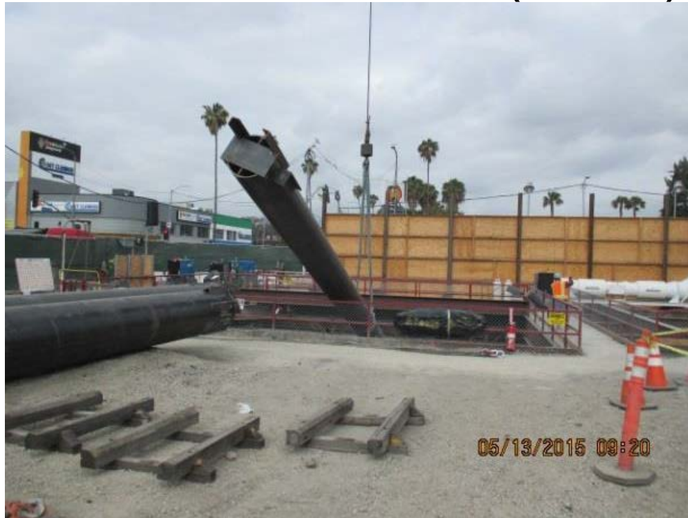
Hoisting Strut Down the Expo Shaft.
