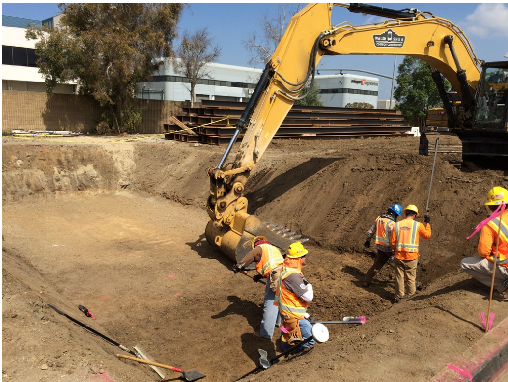
111 th Street Underpass Abutment 2 Footing Excavation.
