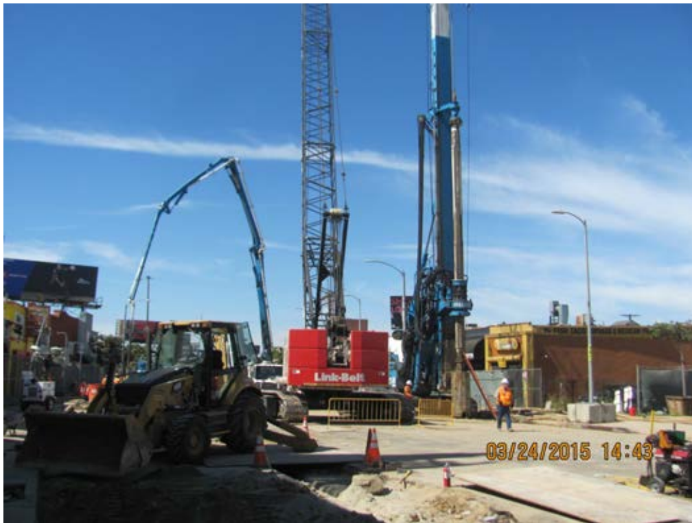
Vernon Piling Operation.
