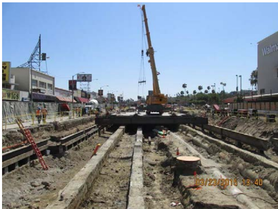
MLK Decking Operations.
