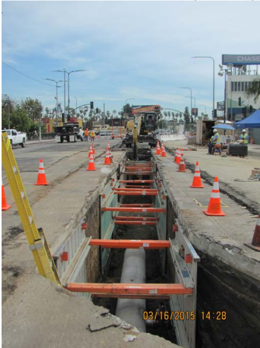
DWP Relocation of 24" Waterline at Vernon.
