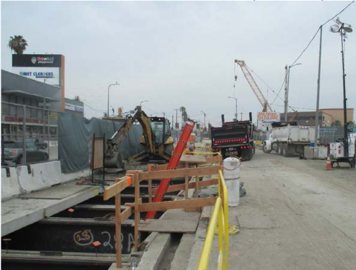
Soil Removal at Beam 32-33 at Exposition Station.
