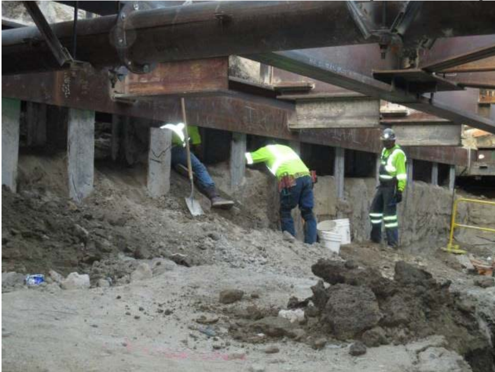
Removing Soil and Placing Lagging on the north wall of the Expo Station.
