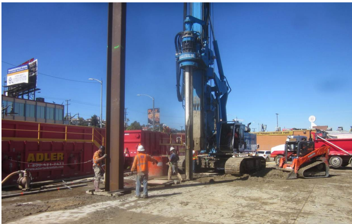
Soldier Pile Drilling and Beam Placement for Excavation Support at Vernon Station.
