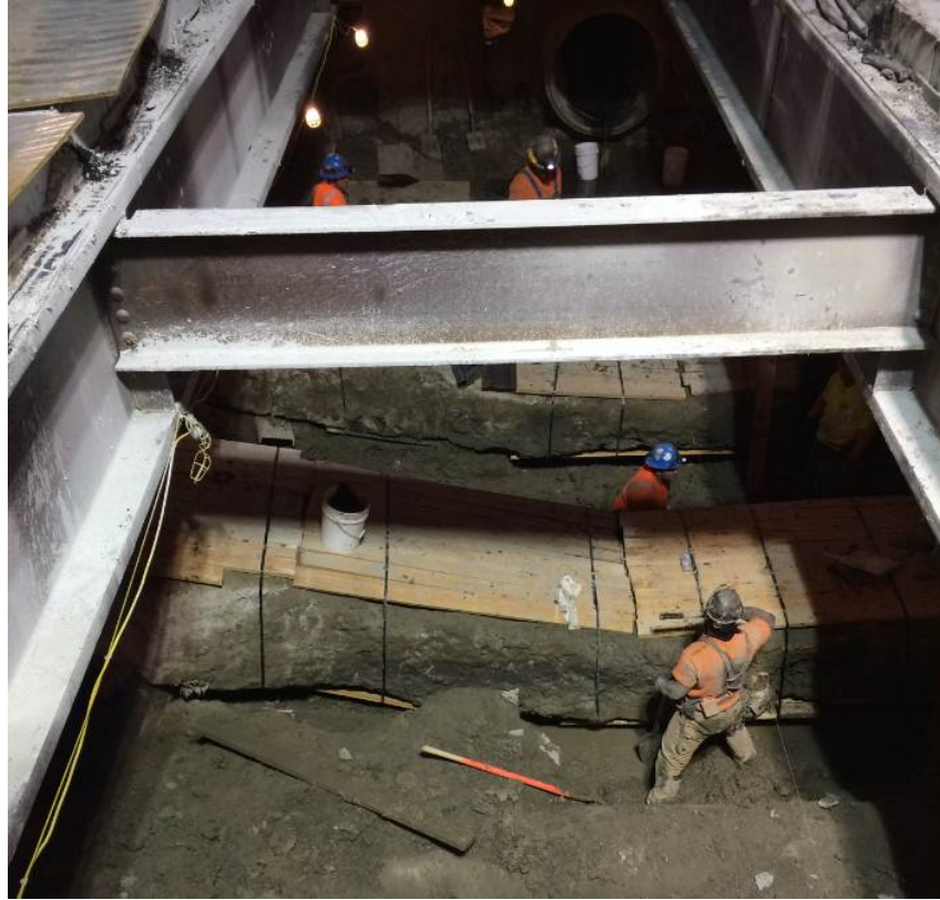
Expo Station Utility Support.
